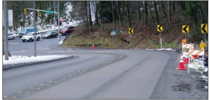
The challenging road geometry of this intersection in the City of Bellevue, WA made HFST a good solution for reducing run-off-road crashes. Source: FHWA
