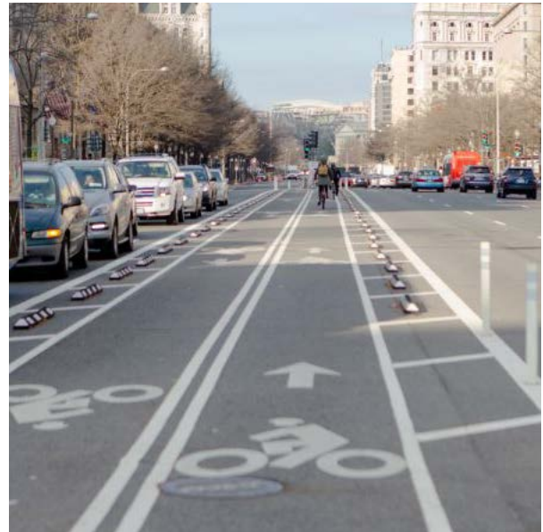
A two-way bicycle lane facility. (Source: FHWA)
