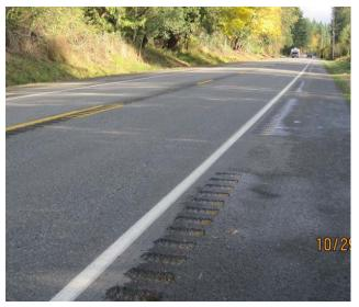
This photo depicts both center line as well as shoulder rumble stripes. Bicycle gaps permit bicyclists using the shoulder to cross the rumble strip area without striking the milled pattern. Source: FHWA
