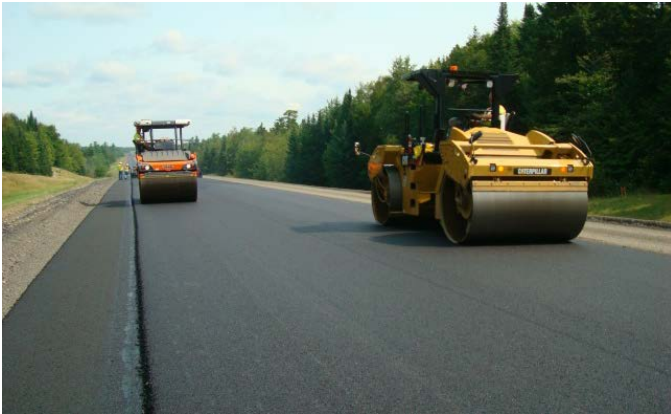
Double drum steel wheel vibratory roller machines smooth a newly paved roadway. Photo courtesy of Transtec, Inc.
