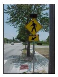
Drivers generally do not yield the right-of-way to pedestrians in marked crosswalks at uncontrolled sites. One alternative to in-roadway signs and yellow flashing beacons is to add yellow LED Rectangular Rapid-Flashing Beacons (RRFB) to pedestrian warning signs. These LED RRFBs are similar in operation to emergency flashers on police vehicles. The photo to the left shows an RRFB mounted below a W11-2 pedestrian warning sign at a crosswalk.
