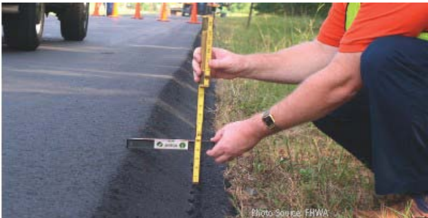
Photo Source: FHWA
