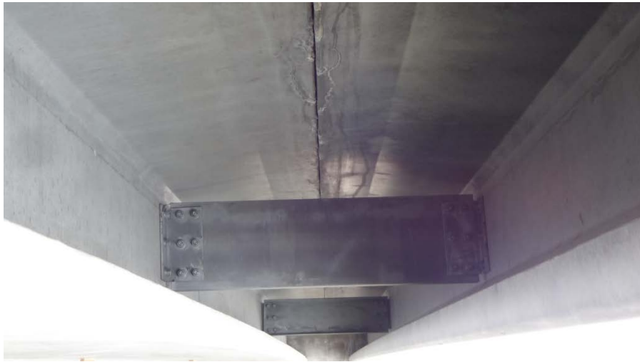
Figure 2.3: Diaphragm Connecting Girders of the Bridge
