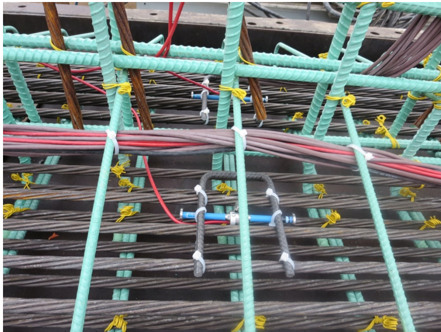
Figure 2.13: Strain Gauge placed in the Web
