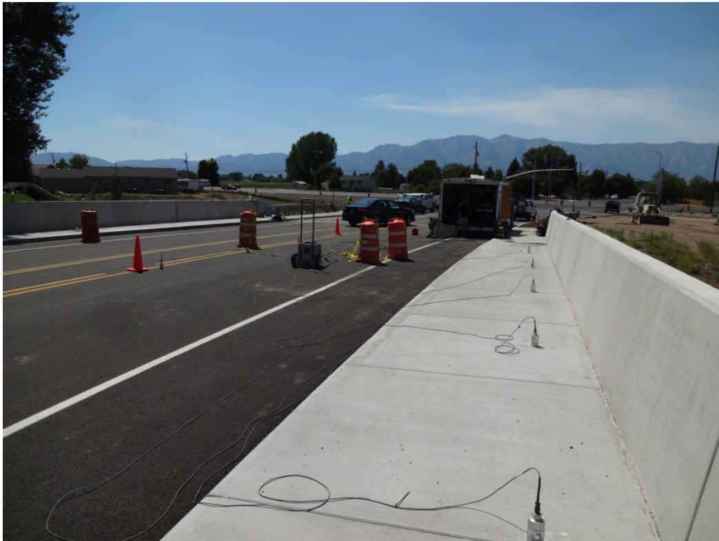
Figure 3.7: View along the North Side of the Bridge during the Test
