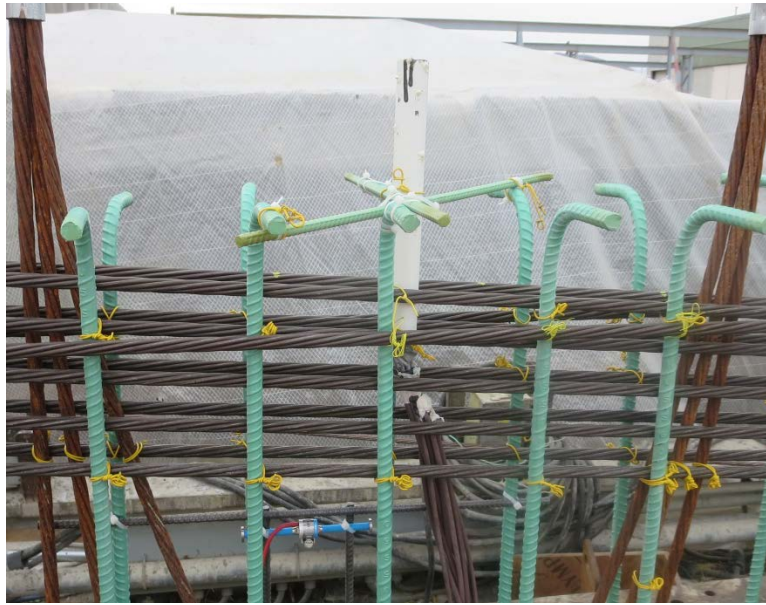
Figure 2.14: Thermocouple Placement during Construction
