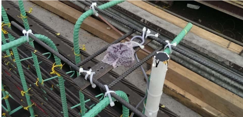
Figure 2.15: Embedded Accelerometers during Construction
