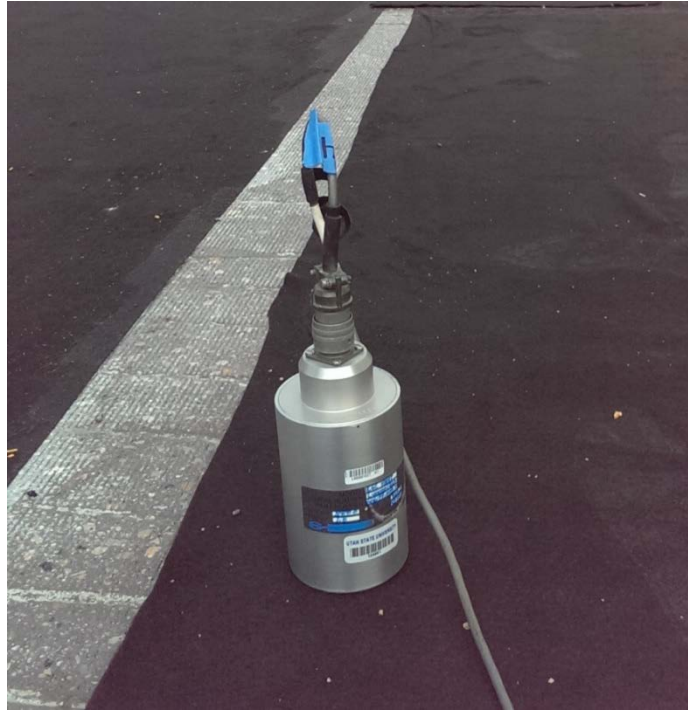
Figure 2.16: Velocity Transducer on the Bridge prior to Asphalt Installation
