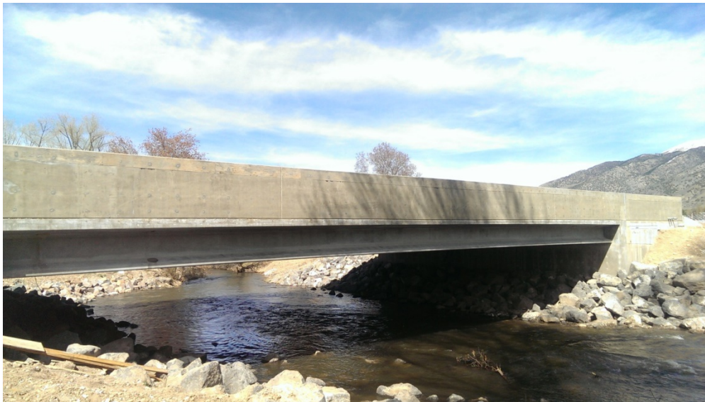
Figure 2.1: Elevation View Looking North
