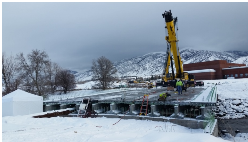
Figure 2.2: Girder Placement during Construction (Ira Tibbits, personal communication, Oct. 18, 2016)
