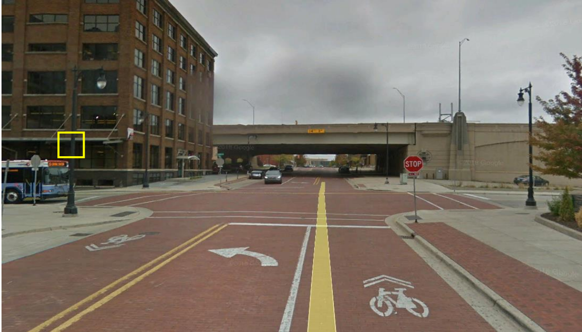
Video camera location: Light pole
