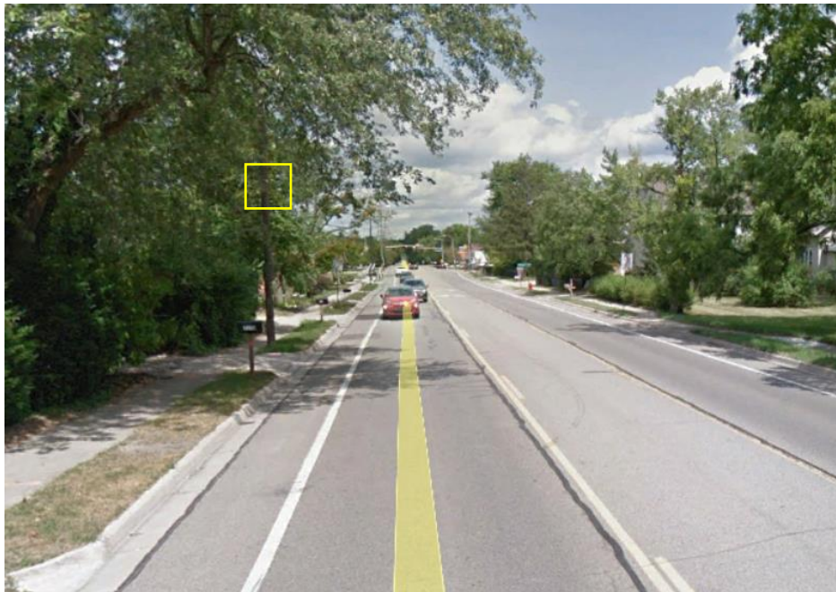
Video camera location: Electric pole
