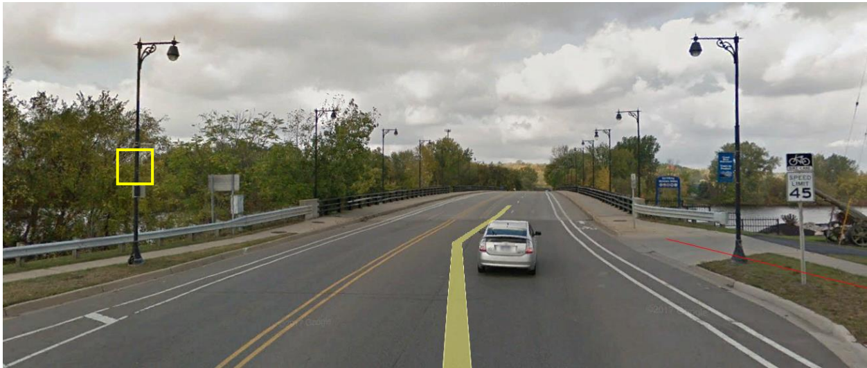
Video camera location: Light pole
