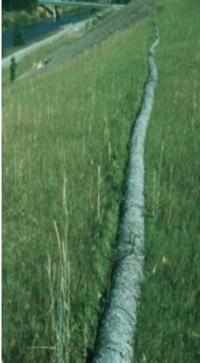
Fiber rolls intercept runoff and remove sediment (BMP SC-5).
