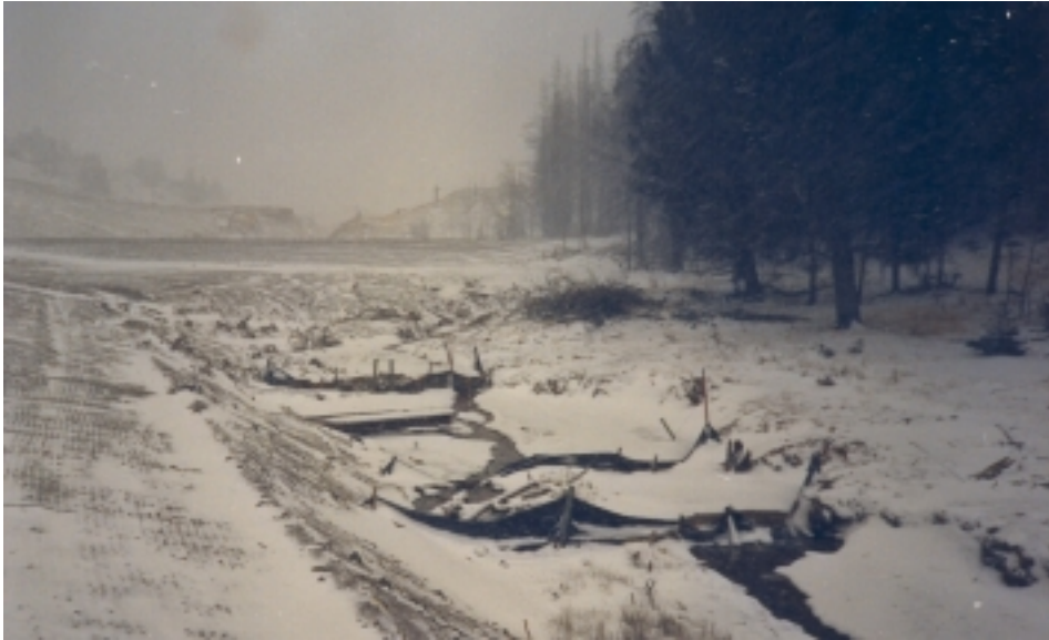
Winter conditions such as heavy snow and ice can cause BMP failure.
