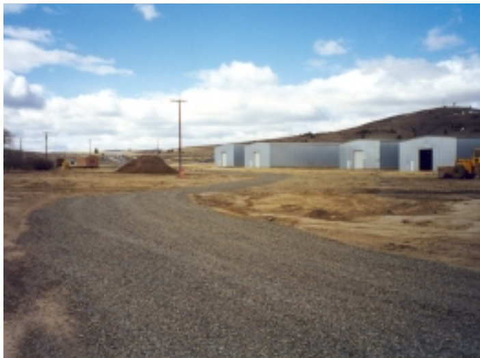
Stabilized construction roads limit dust generation and off-site tracking of soil (BMP TC-2).
