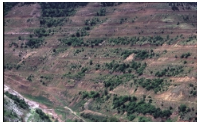
Terraced slopes help reduce velocities and allow deposition of sediment on the terraces. Steep slope revegetation can be a difficult task (BMP SS-13).
