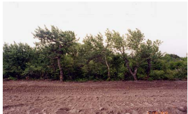
Preserving existing vegetation within and adjacent to construction sites has a positive impact on erosion and sediment control (BMP SS-2).
