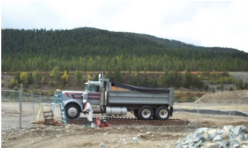
Washing tires at construction site outlets reduces off-site tracking of soils that they may end up in waterways (BMP TC-3).
