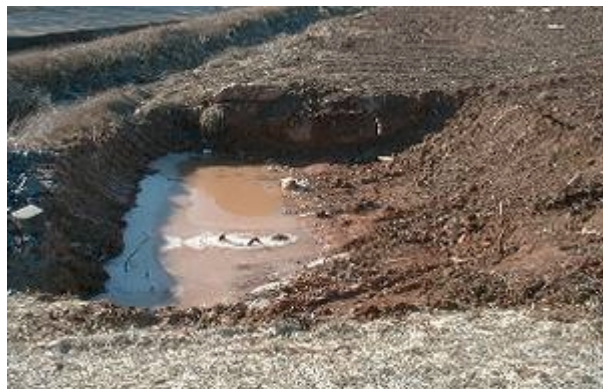
Sediment traps are used to collect sediment laden runoff from disturbed areas on construction sites (BMP SC-3).
