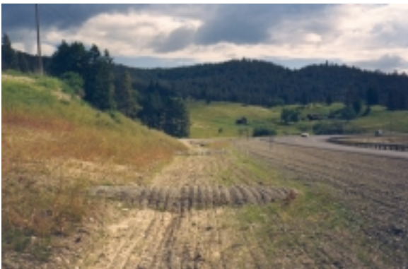
Check dams provide minor water ponding and removal of sediment (BMP SC-4).
