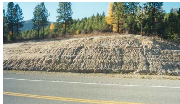
Water erosion from bare slopes is a major source of erosion.
