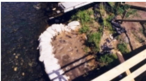
Sandbag barriers are used for slowing the flow of sediment laden water or to divert water flows (BMP SC-8).
