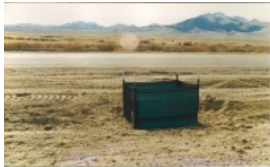
Silt fencing is one method of providing storm drain protection during construction (BMP SC-10).
