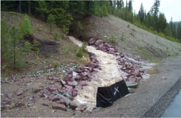
Rock Lined channels are a method of conveying discharges with a minimum of soil erosion (BMP SS-9).
