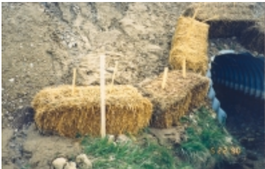
Straw bale barriers used to intercept runoff and remove sediment (BMP SC-9).
