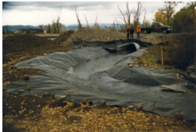
Synthetic liners can be used to minimize soil erosion during construction (BMP SS-7).
