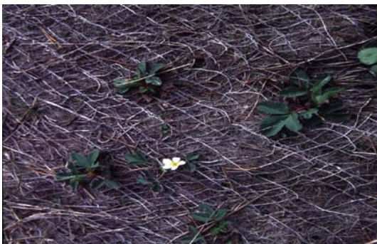
Erosion control mats are often used to prevent erosion and aid in the reestablishment of vegetation (BMP SS-7).
