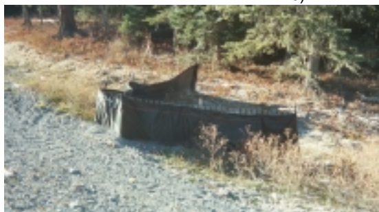
Silt fencing is also used to protect culvert inlets and outlets from sediment (BMP SC-1).
