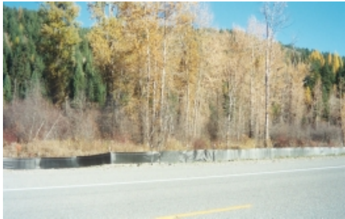
Silt fencing is a commonly used sediment control BMP (BMP SC-1).
