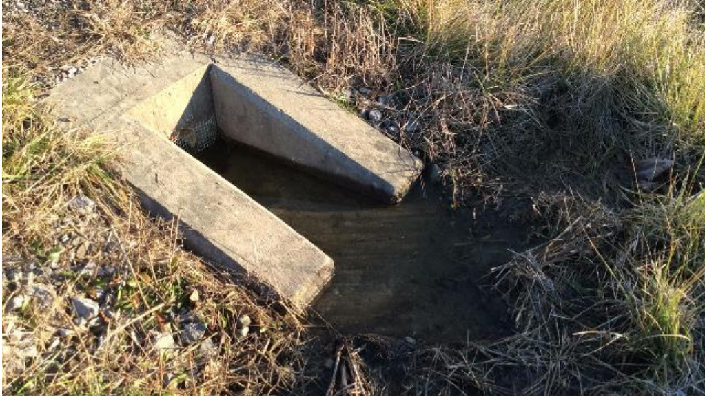
Figure 7 Outlet Waterway and Outfall Waterway Holding Water
