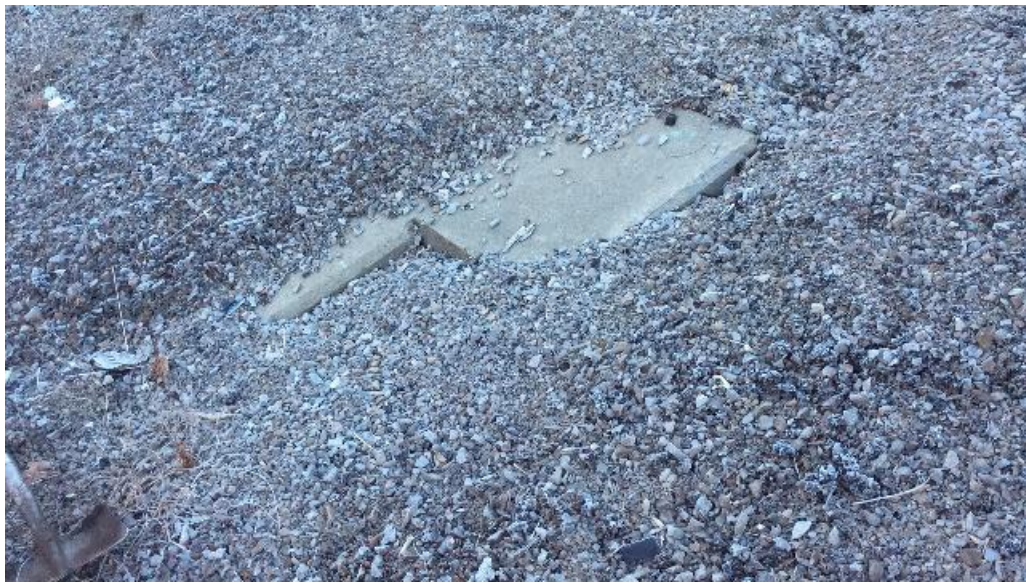
Figure 6 Waterway Completely Inundated
