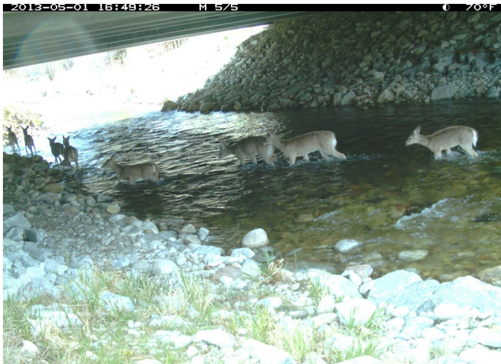
Figure 60. US 93 mp 50.3 Blodgett Creek Bridge, 2.7 (H) x 25 (W) x 27.4 (L) meters, 9 x 82 x 90 feet, Openness Ratio (meters) 2.4.
