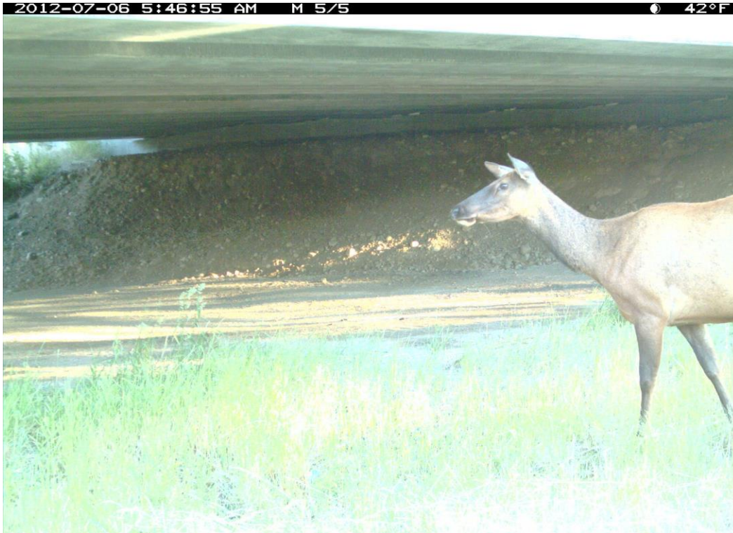
Figure 44. US 93 mp 69.7 Dawn's Crossing Bridge, 4 (H) x 135 (W) x 24 (L) meters, 13 x 115 x 79 feet, Openness Ratio (meters) 5.8.
