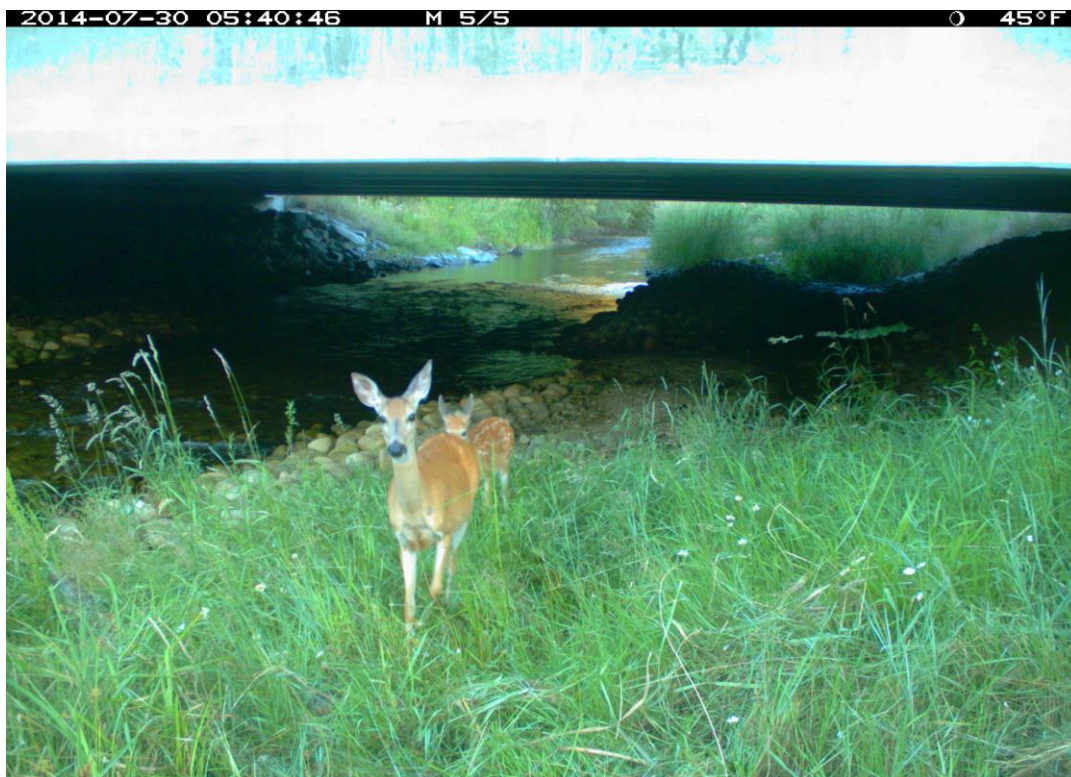
Figure 53. US 93 mp 59.7 Sweathouse Creek Bridge, 2.2 (H) x 25.5 (W) x 29.3 (L) meters, 7.2 x 84 x 96 feet, Openness Ratio (meters) 1.9.
