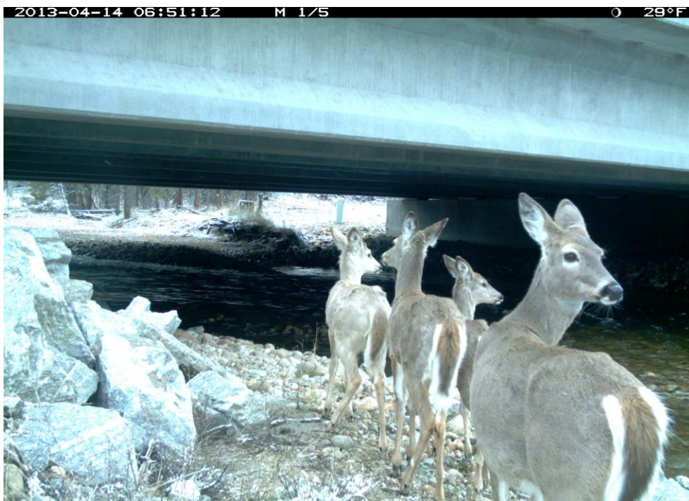
Figure 51. US 93 mp 61.6 Big Creek Bridge, Southeast Side.
