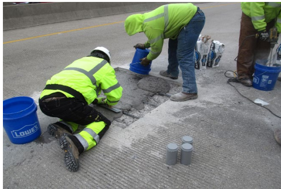
(a) Placing Phoscrete
