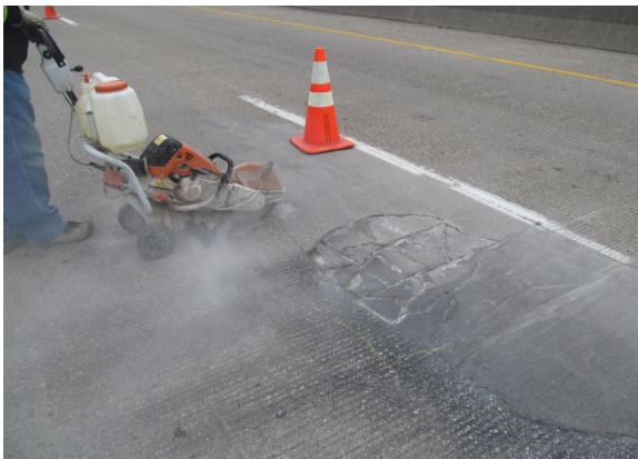
(a) Saw cutting repair edge
