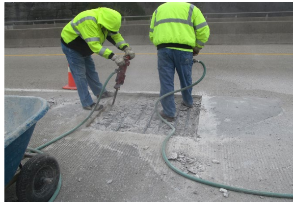
(b) Chipping Concrete
