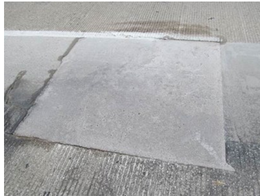
Figure 18 Repaired Patch One Year Later
