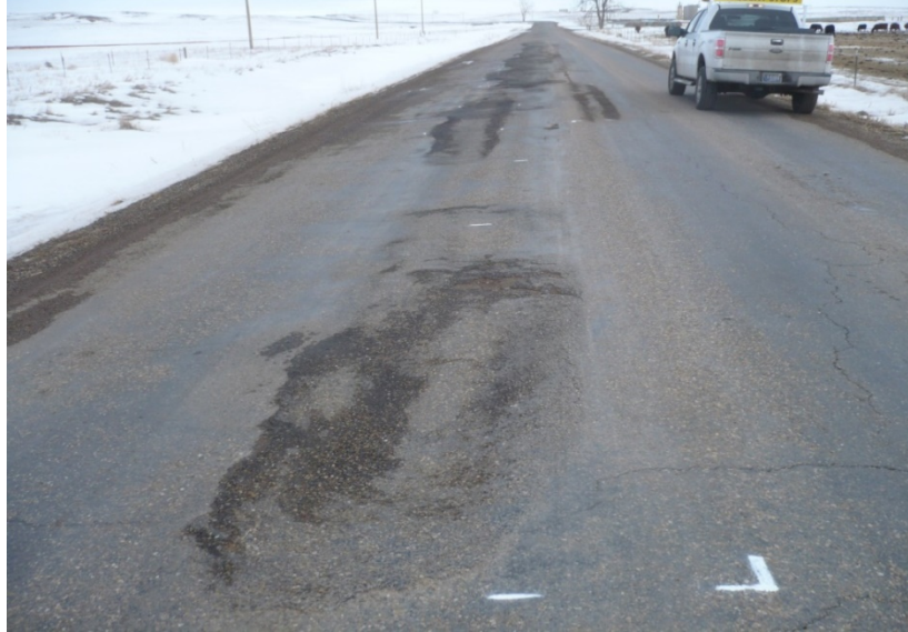
FIG. 17. Heavy load damage to green soil cement in left lane. Right lane was exposed to the same loading, but had three days of additional cure.
