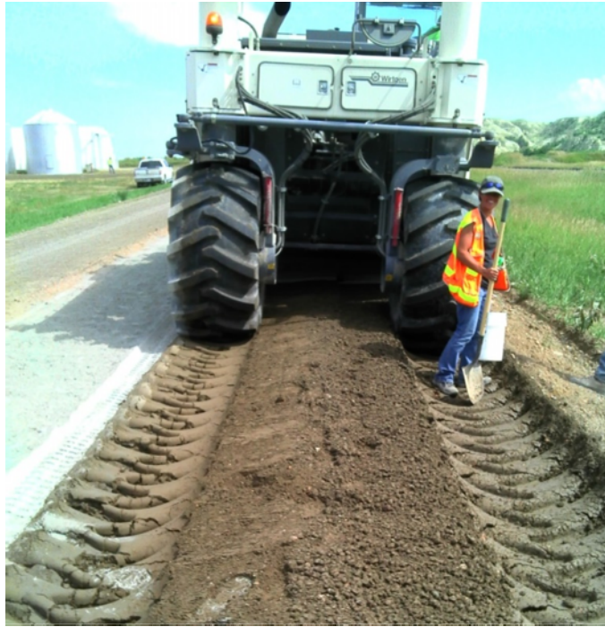
FIG. 27. Good pulverization on left and bad pulverization on right.
