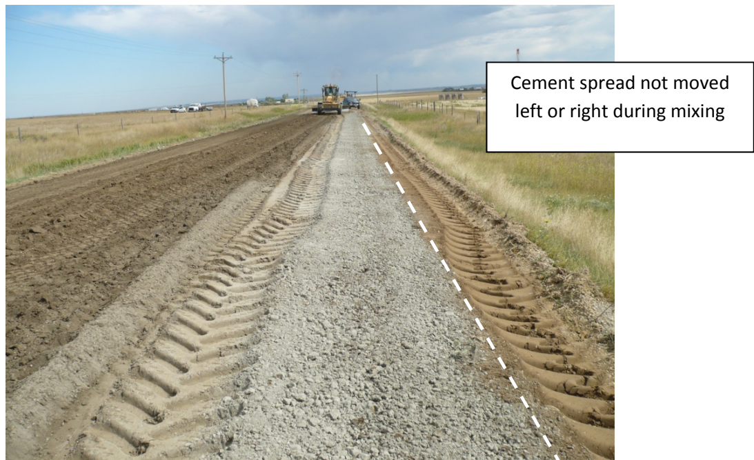
FIG. 25. Cement is not moved left or right during mixing.
