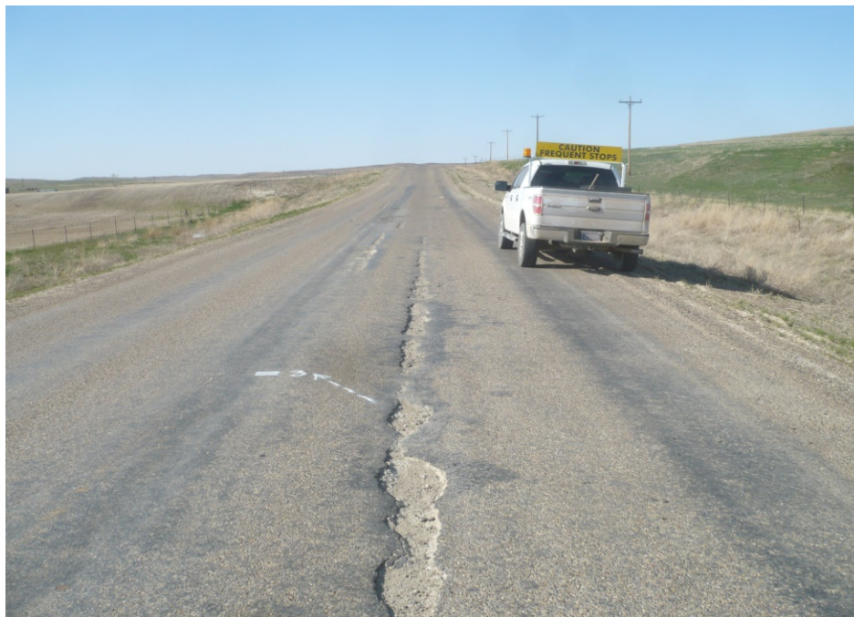
FIG. 15. Otta seal BST “pot hole” area where stopped traffic pulled BST off soil cement surface, CR 146W.
