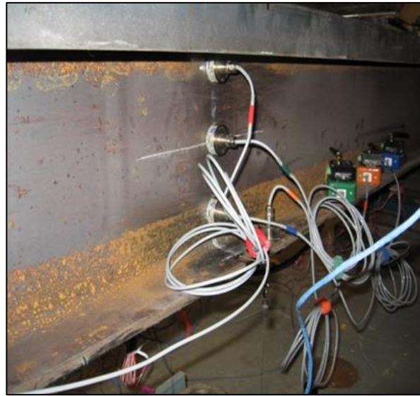
Fig. 3 Magnetic gauges mounted on steel beam
