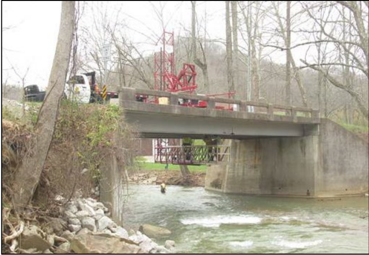
Fig. 8 Attaching strain gauges from work platform
