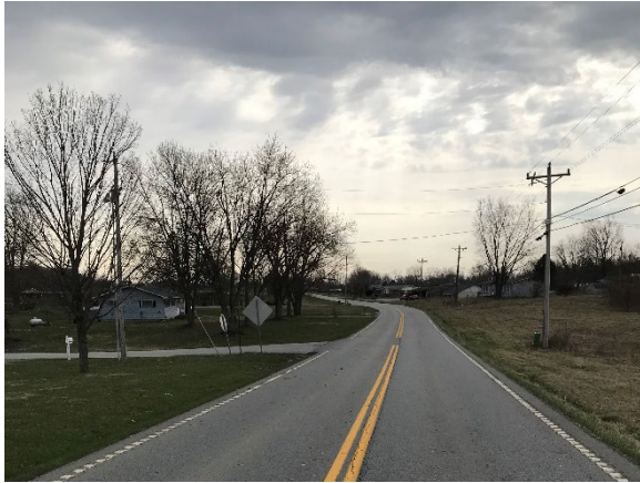
Figure 13. Overview of Roadway
