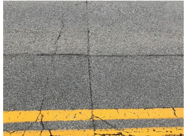
Figure 18. Transverse Cracking
