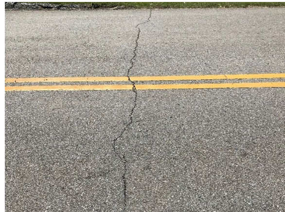
Figure 30. Transverse Cracking
