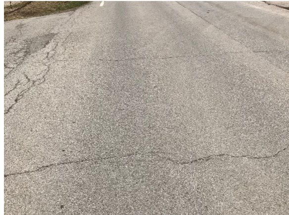
Figure 44. Transverse Cracking
