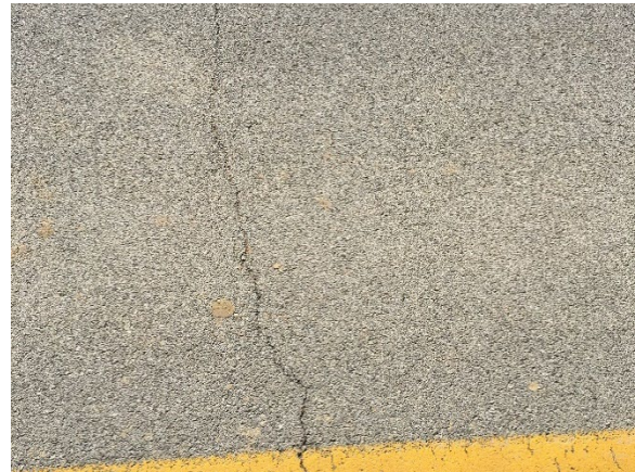
Figure 36. Transverse Cracking
