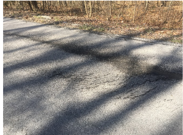
Figure 38. Shoving Pavement
