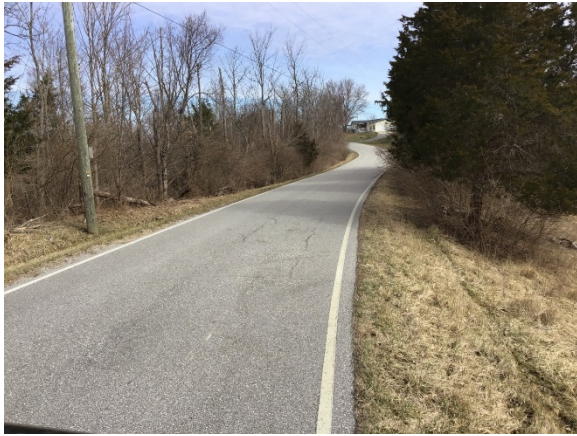
Figure 5. View of Roadway
