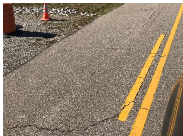
Figure 32. More Cracking
