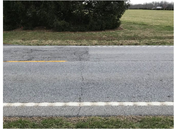
Figure 14. Transverse Cracking
