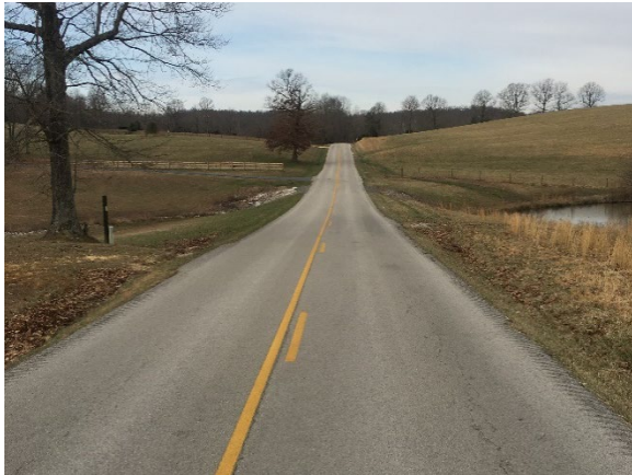
Figure 33. View of Roadway
