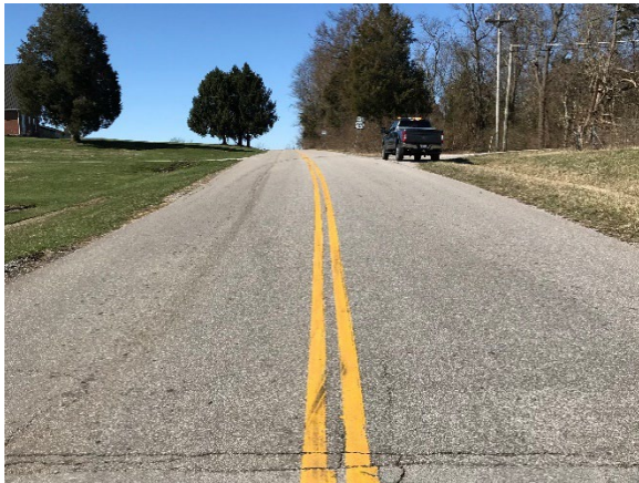
Figure 29. View of Roadway
