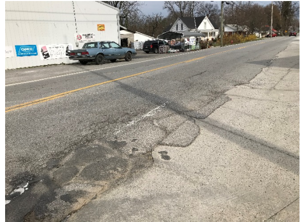
Figure 46. Patching Along Outside Edge
