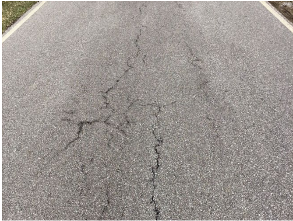
Figure 7. Moderate Cracking Middle of Lane
