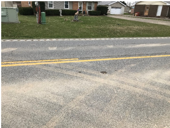
Figure 15. Longitudinal Cracking
