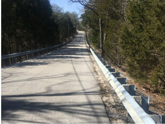
Figure 37. View of Roadway
