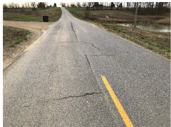
Figure 28. Transverse Cracking
