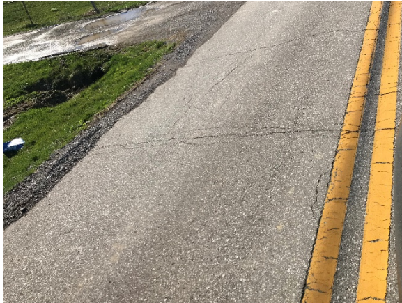
Figure 3. Transverse Cracking
