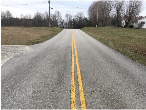
Figure 9. Overview of Roadway
