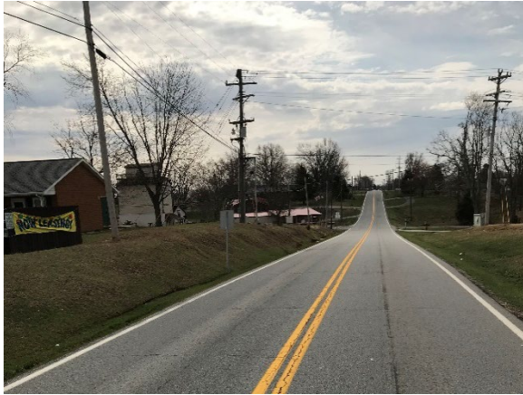
Figure 17. View of Roadway
