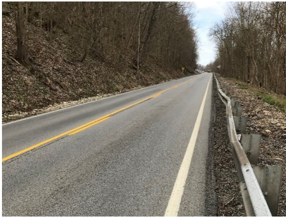
Figure 21. View of Roadway
