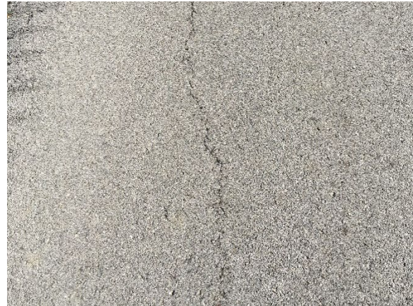
Figure 34. Longitudinal Cracking
