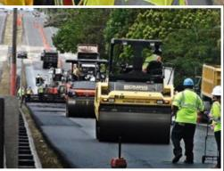
Professionals from the public and private sectors collaborate on using innovative technologies such as warm-mix asphalt. Inset: The Puerto Rico Highway and Transportation Authority is using warm-mix asphalt to cut fuel consumption and fumes on paving projects. **Design-Build Cuts Years and Millions of Dollars From Missouri Project**
