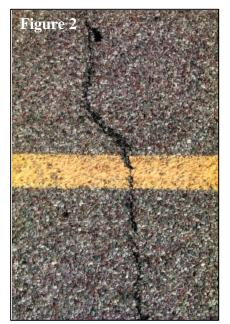
Average transverse cracking per mile (CPM) is 23 with a standard deviation of .99. Note that almost all transverse cracking observed was at milepost 28. Three transverse cracks
