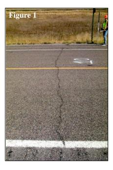
across both lanes, less than ¼? within the 300?data collection site. This amount of cracking is considered an anomaly and not representative of the entire project that has (at this time) exhibited minimum cracking. Figure 1 shows an example of one of the low-severity
