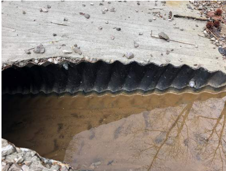
Figure 8 Mitered Pipe End Secured to Headwall
