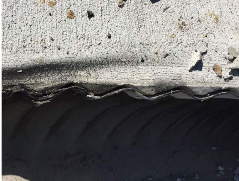
Figure 4 Separation Between Headwall and Pipe End
