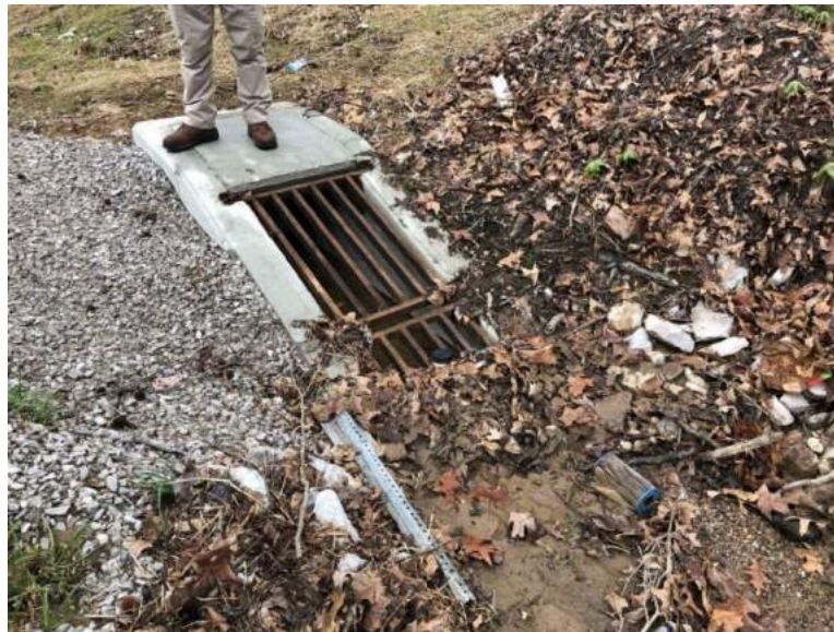
Figure 10 Safety Type Box Inlet Grate Blocked
