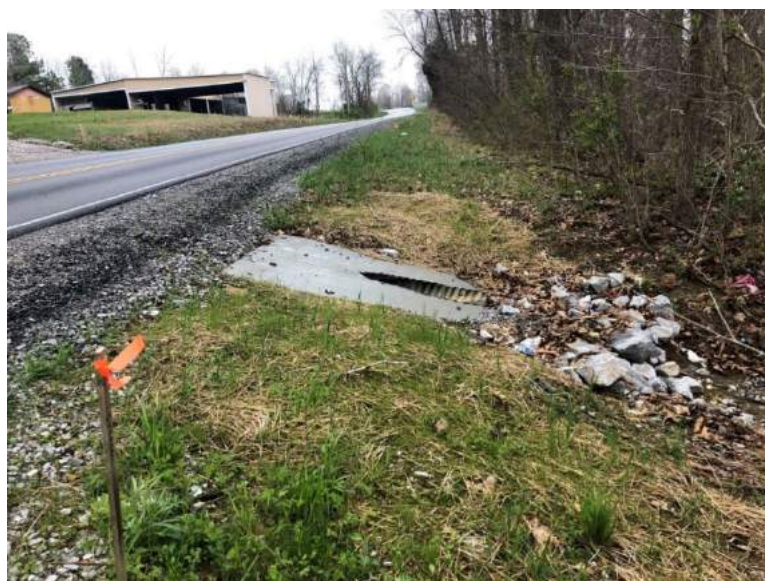
Figure 7 New Headwall and Improvements to the Clear Zone
