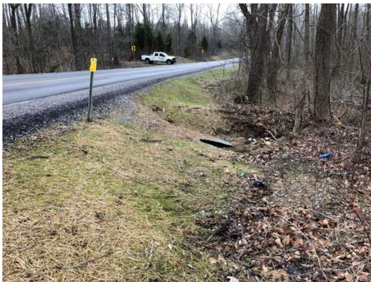
Figure 9 Depression Above Pipe
