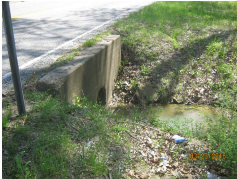
Figure 6 Existing Headwall
