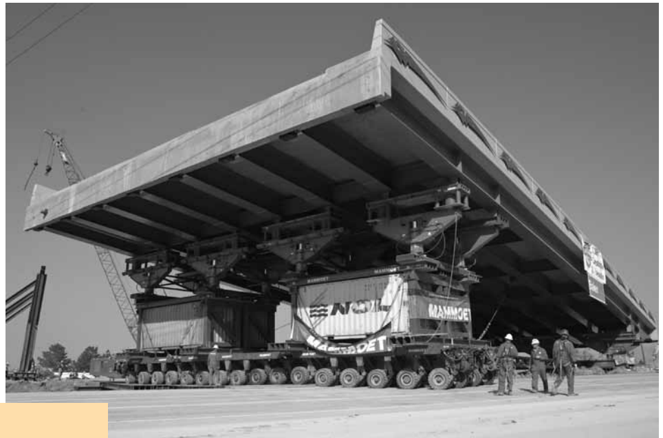
The Utah Department of Transportation installed the prefabricated superstructure of the 4500 South bridge over I-215 in Salt Lake City in 2007.
