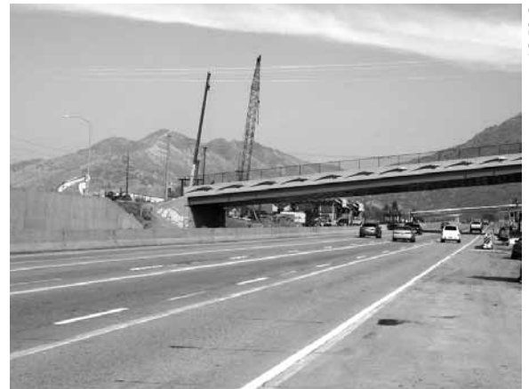
Following installation of the new bridge, I-215 reopened to traffic after a single weekend of work.
