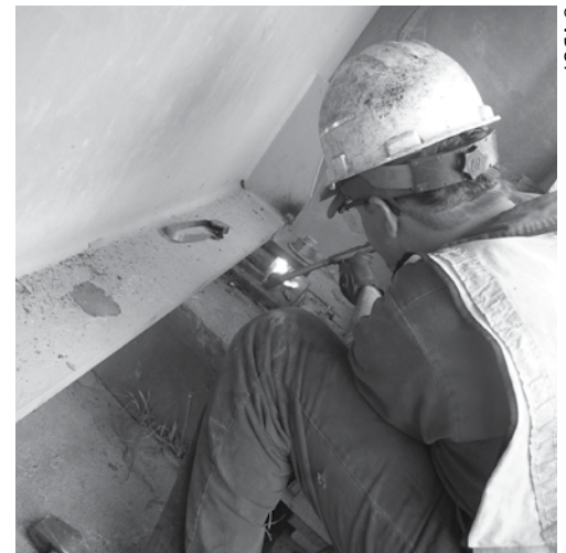
Work is done on a bearing device to facilitate the proper expansion and contraction of a bridge.
