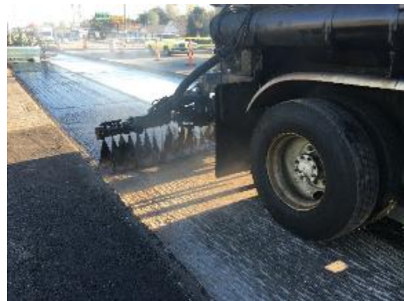
Figure 11 Applying Tack Coat as Adhesive
