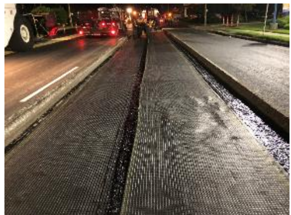
Figure 26 View of Installed Fabric
