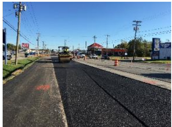
Figure 14 Compaction of Base Course
