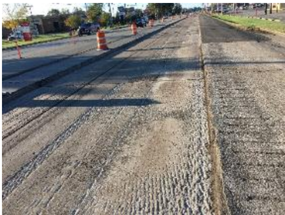
Figure 10 Pavement Prepped for Fabric
