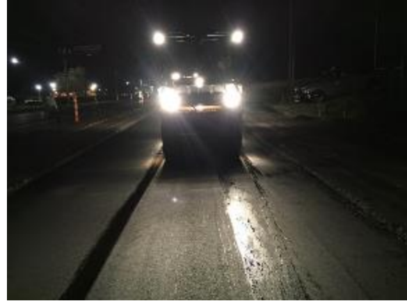
Figure 8 Compaction of RCRI
