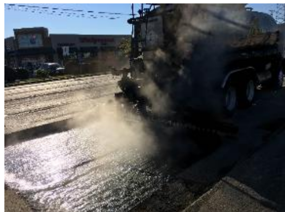
Figure 18 Applying Tack Coat as Adhesive
