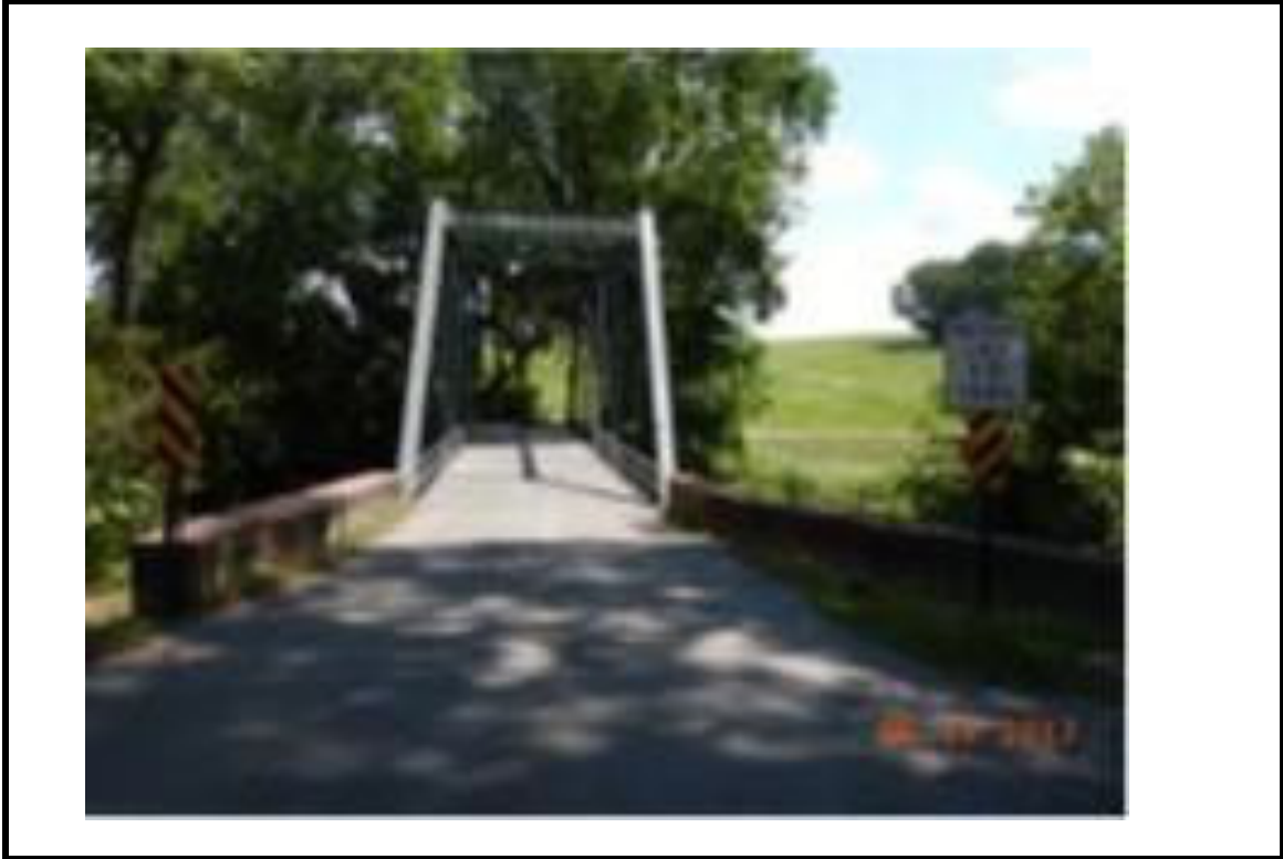
Figure A27: Red River Bridge Summary Sheet
