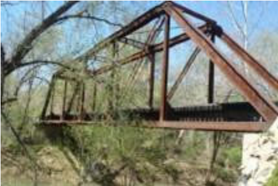
Figure A15: Little Sandy River Bridge Summary Sheet
