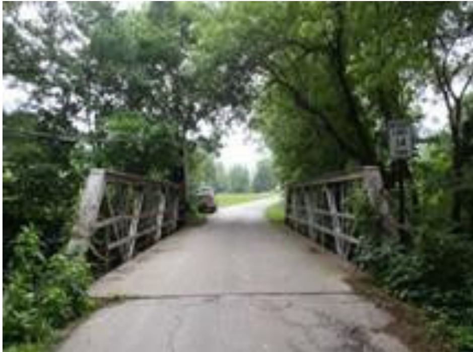
Figure A16: Knob Creek Bridge Summary Sheet
