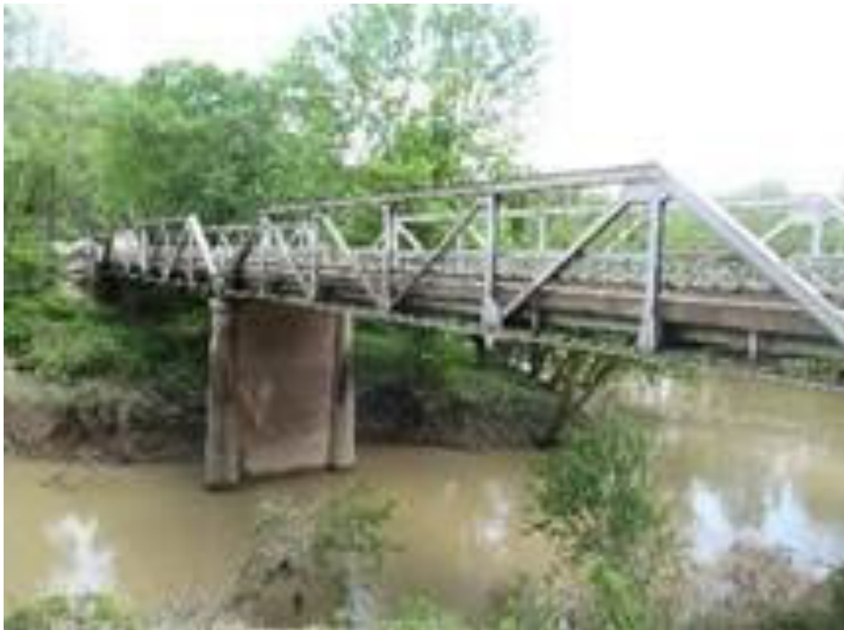
Figure A75: Quicksand Creek Bridge Summary Sheet
