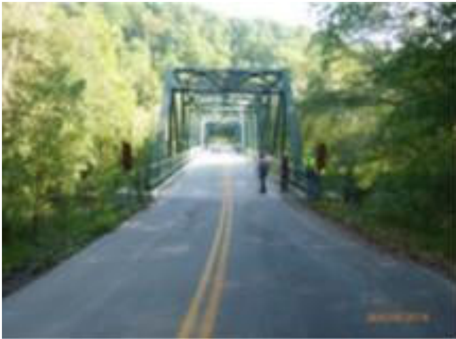
Figure A41: Red River Bridge Summary Sheet
