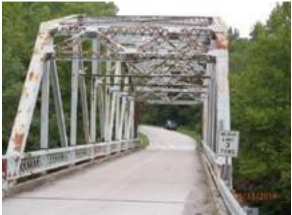
Figure A74: Over Little Sandy Bridge Summary Sheet
