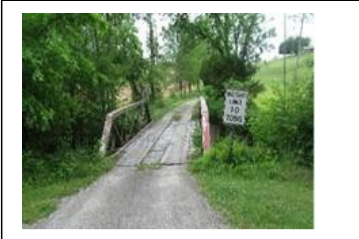
Figure A68: Branch - Rock Creek Bridge Summary Sheet
