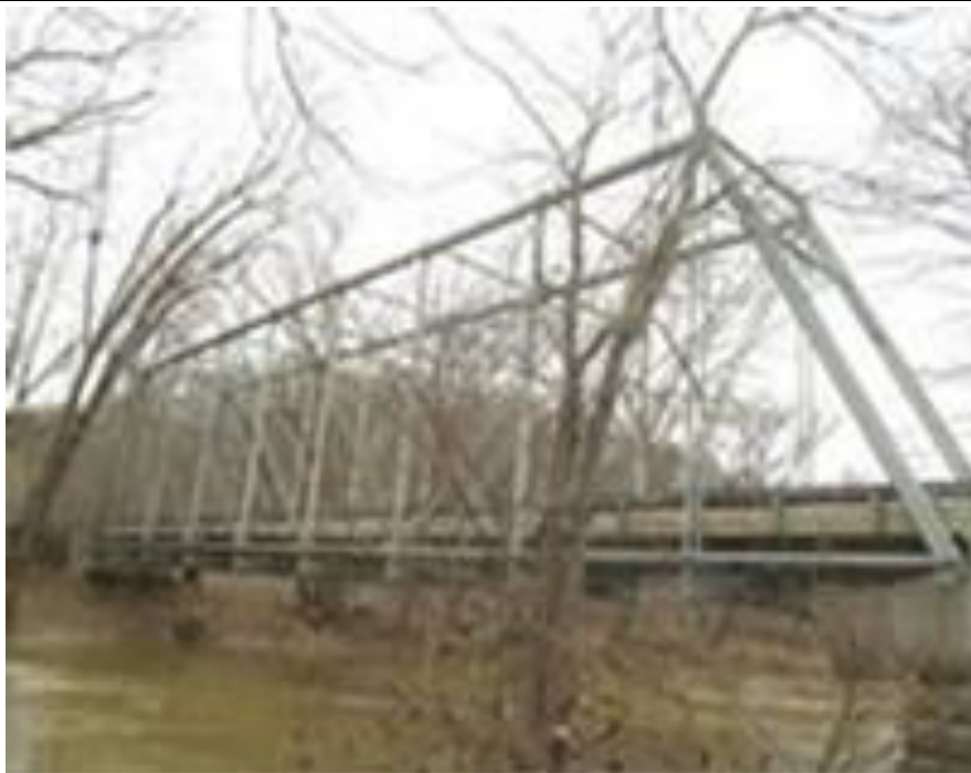
Figure A1: Little Sandy River Bridge Summary Sheet
