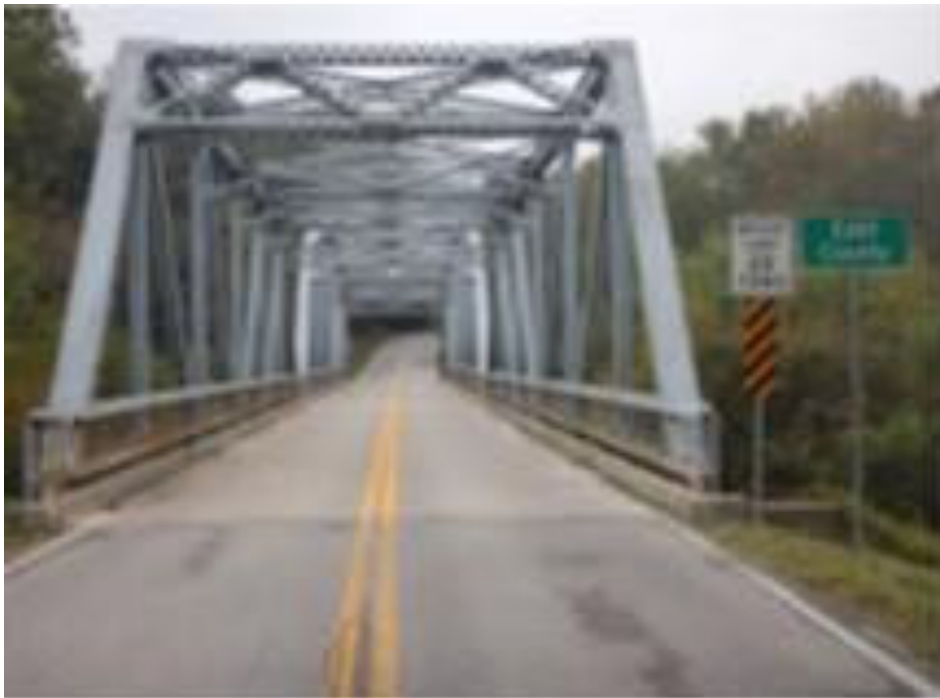
Figure A80: Red River Bridge Summary Sheet
