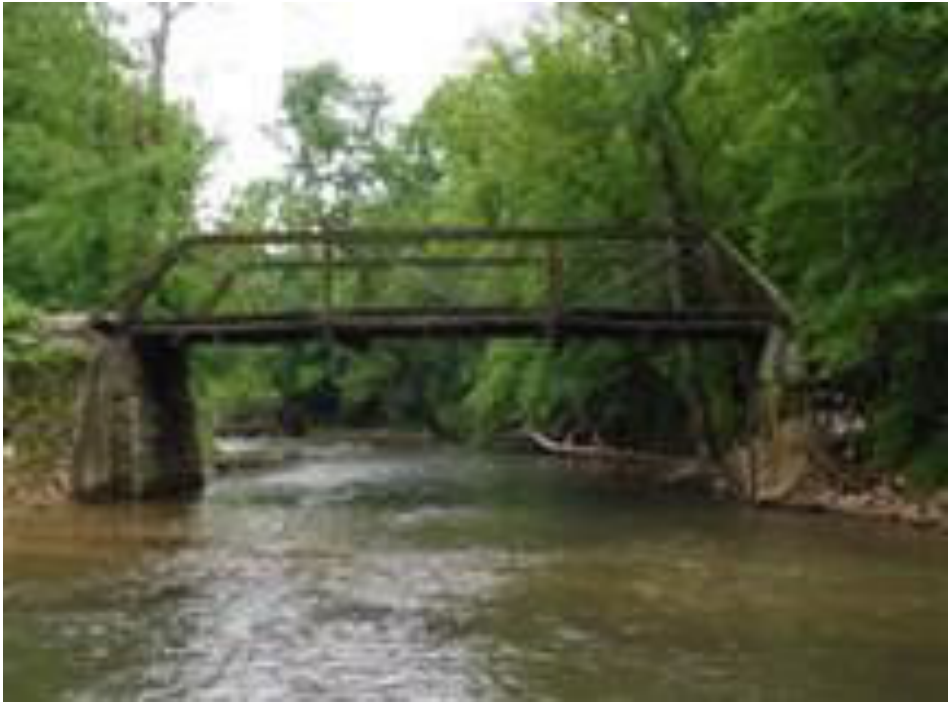
Figure A17: Red River Bridge Summary Sheet
