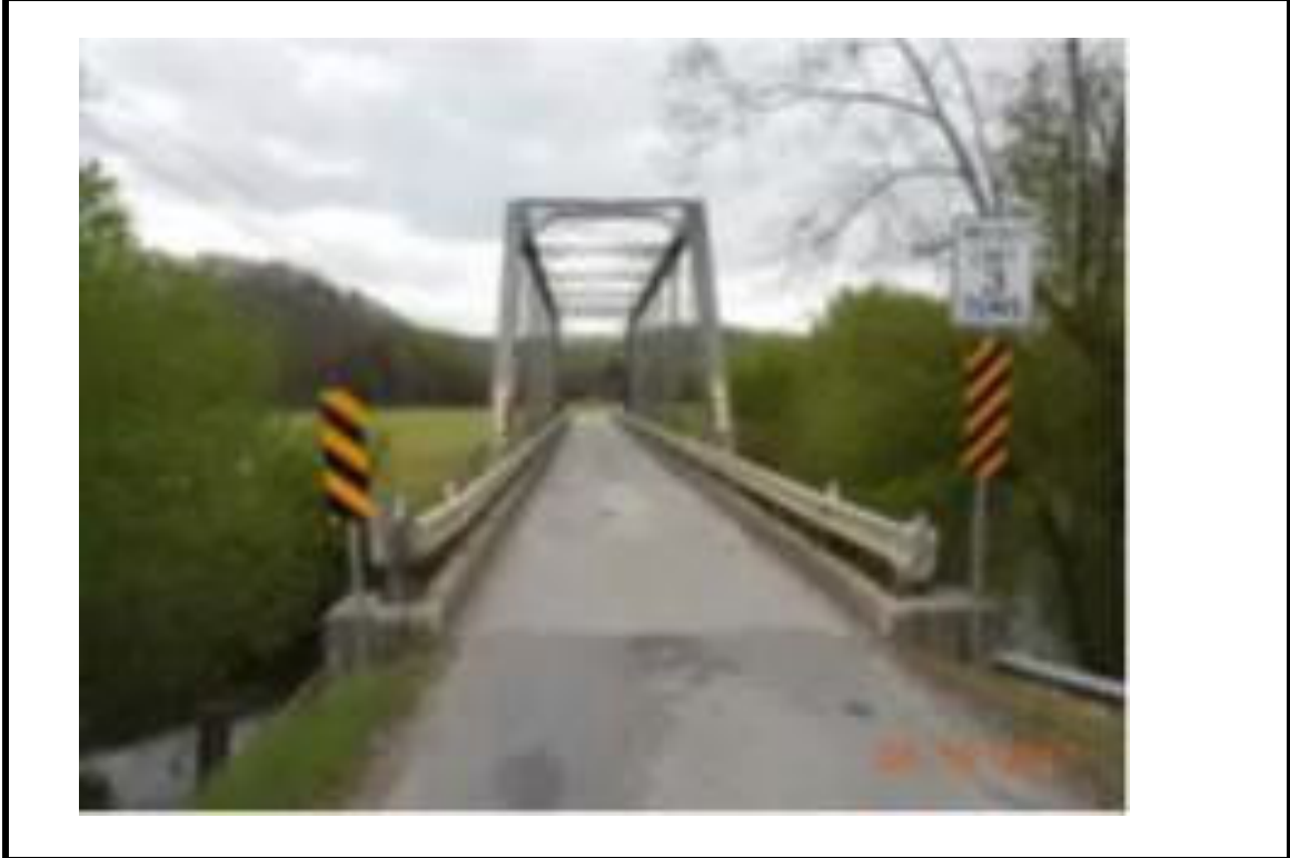
Figure A29: Little Sandy River Bridge Summary Sheet
