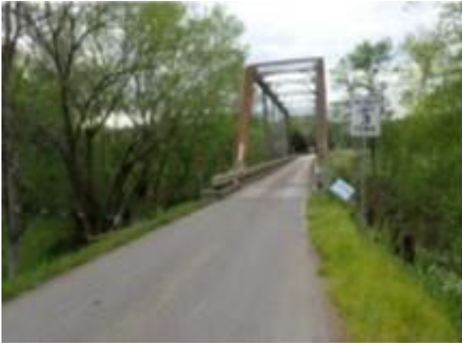
Figure A28: Little Sandy River Bridge Summary Sheet
