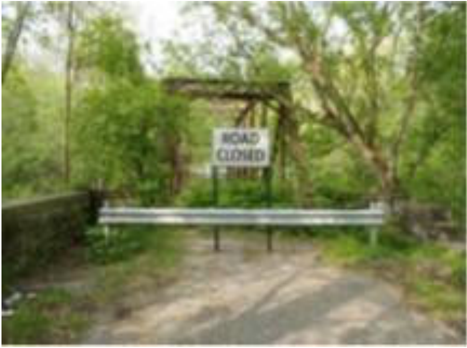
Figure A49: Bluestone @ Triplett Creek Bridge Summary Sheet
