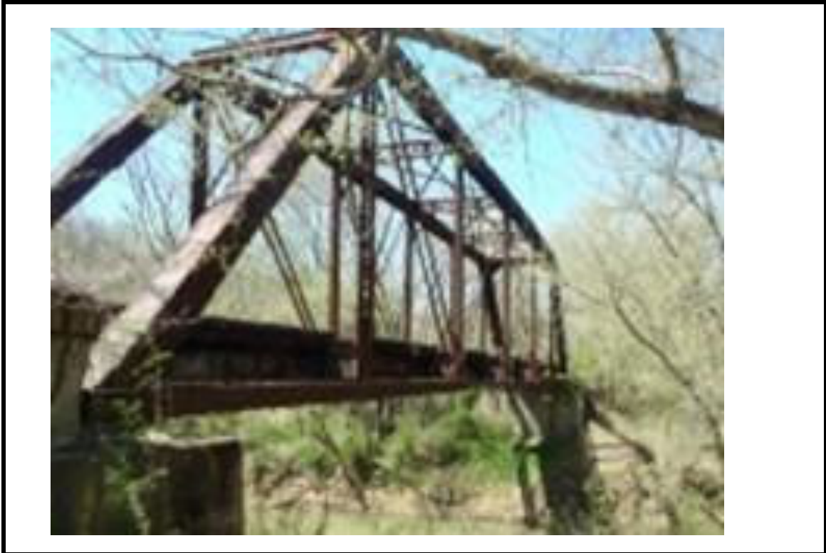
Figure A14: Little Sandy River Bridge Summary Sheet
