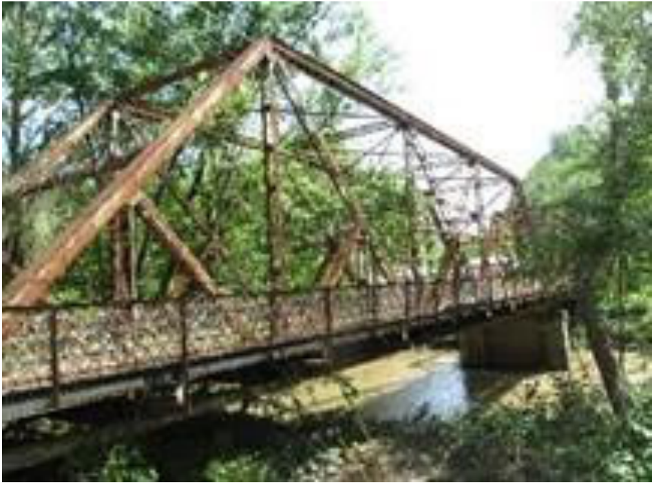
Figure A18: Clover Fork Bridge Summary Sheet
