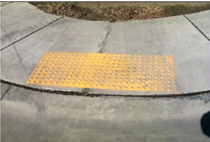
Installation 6B: located on the northwest corner of the intersection 4 th Ave. N. W. and 6 th St. N. W.
