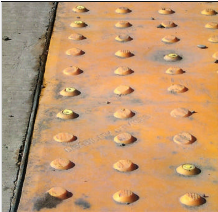
Installation 2: Close-ups of sheared domes and example image of edges losing adhesion.
