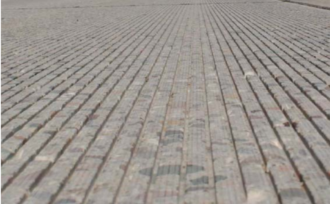
Figure 2-6. Example of NGCS texture characterized by deep grooves with shallow intermediate grooves applied in the longitudinal direction. From (Scofield 2017).
