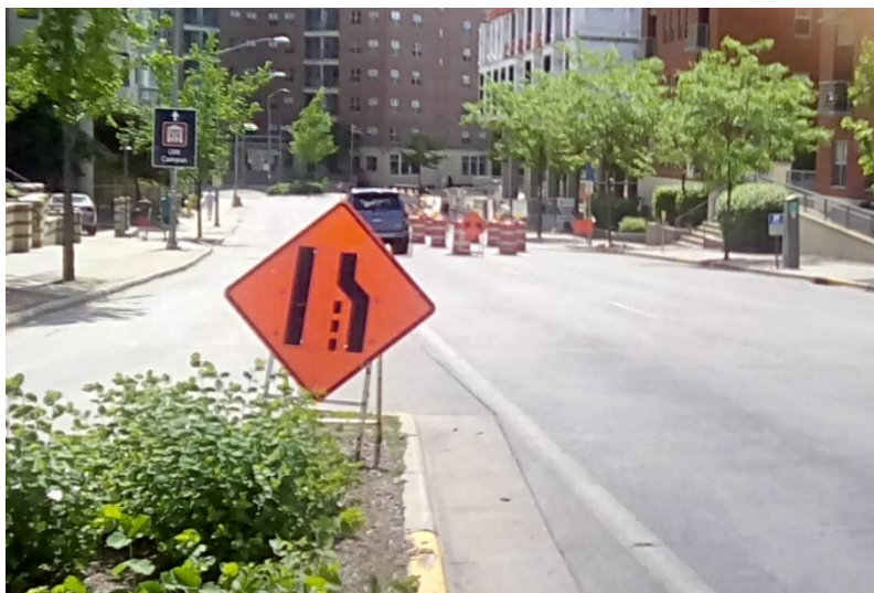
Figure 7. Incorrectly signed center lane closure in Madison, Wisconsin (May 2016)
