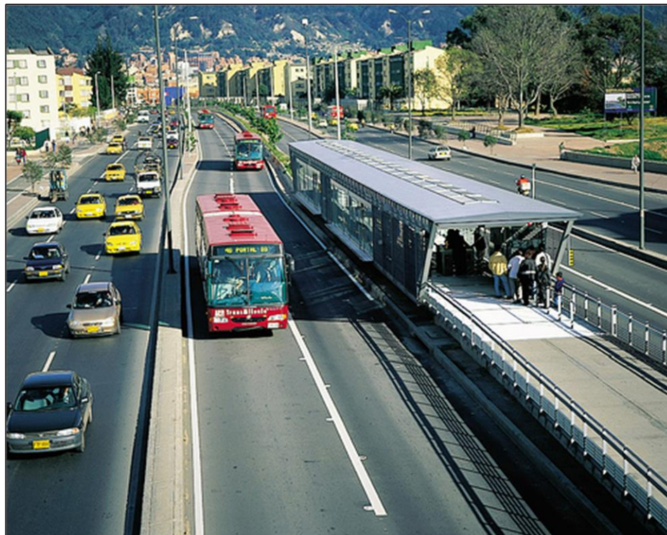
Figure 1.2 - An example of bus rapid transit lanes, Boston, Massachusetts
