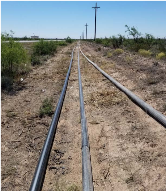
Figure 14. Polyethylene and Lay-Flat Temporary Pipelines.
