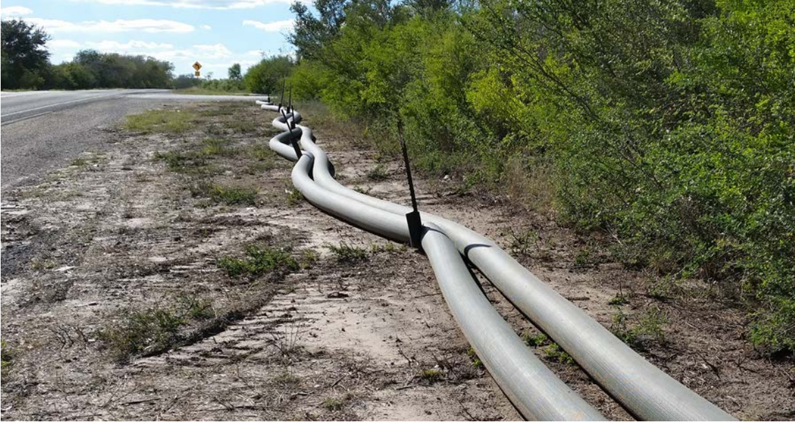
Figure 1. Metal Fence Posts Used to Anchor a Temporary Pipeline in Place.
