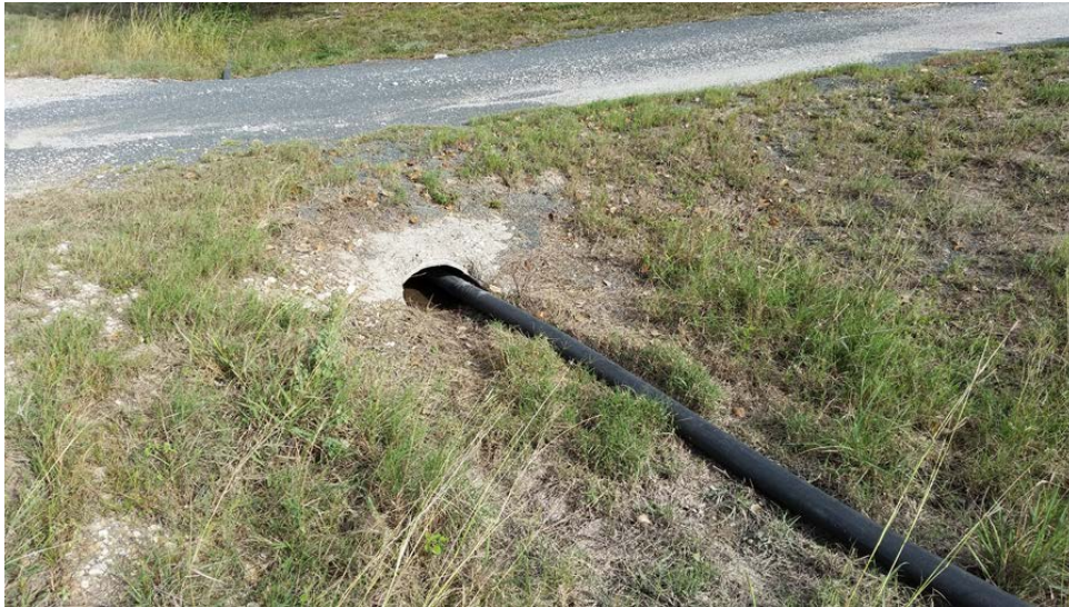
Figure 3. Temporary Pipeline Installed in a Small Diameter Driveway Culvert.
