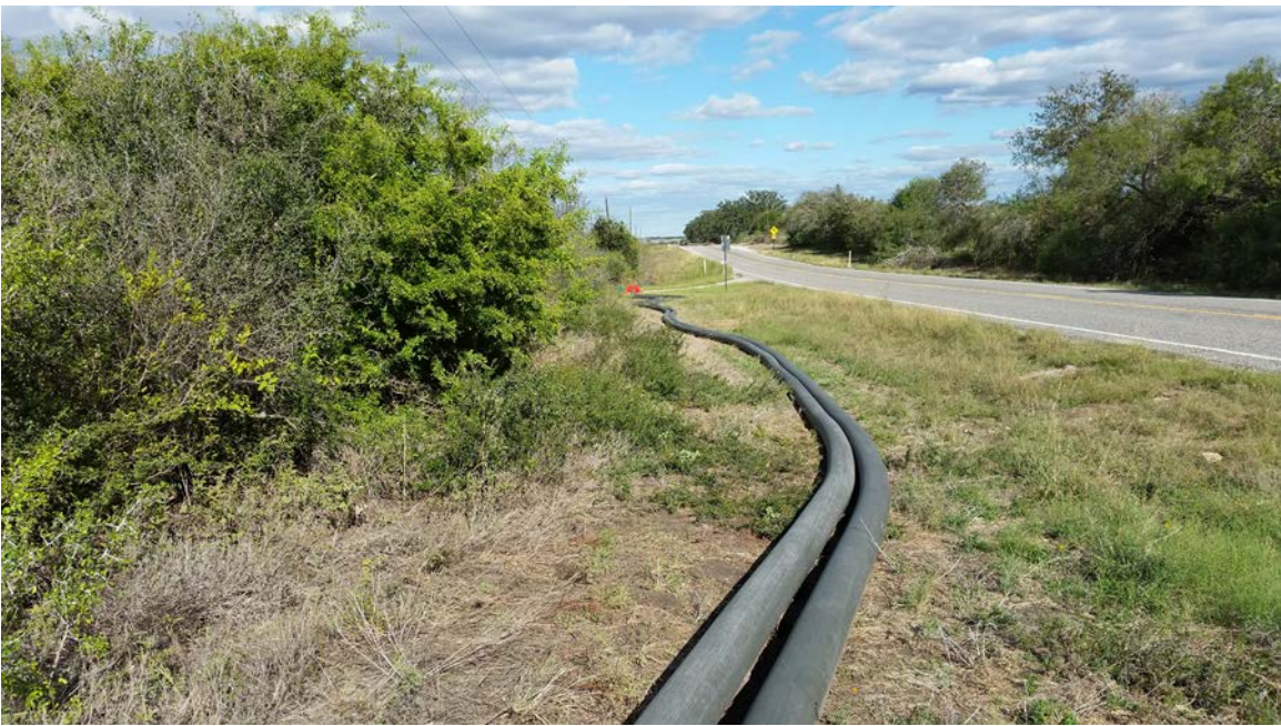
Figure 2. Temporary Pipeline Installation around Vegetation.
