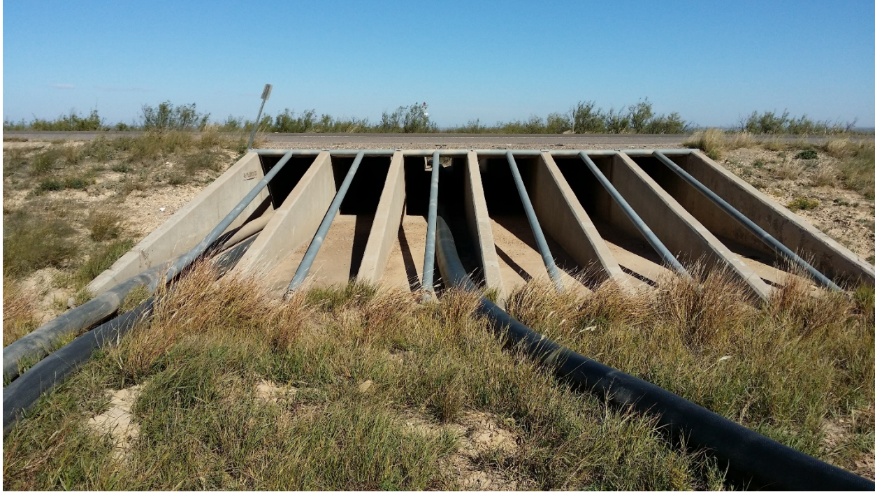
Figure 15. Culvert with Safety End Treatment.
