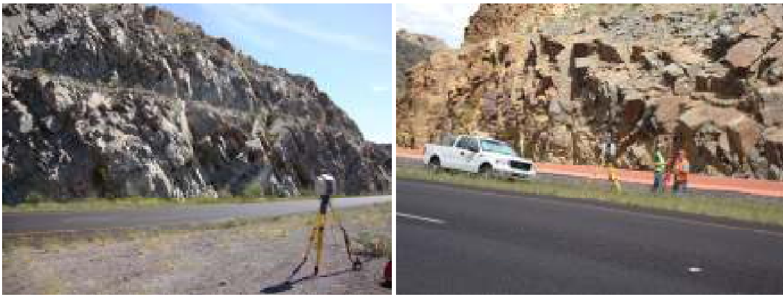
Figure 63. Pictures of Texas site, along with the Leica Scanstation 2 scanner.
