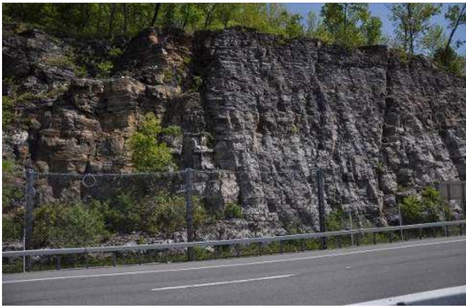
Figure 39. Southern section of rock slope at New York site showing the difference between pre-split (right) and conventional blasting (left).
