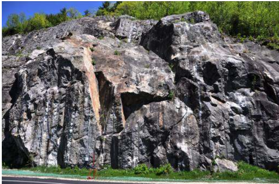
Figure 31. Southern section of the New Hampshire site.
