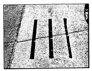
This photo illustrates the placement of the dowel bars in the slots. The dowels are placed on chairs to keep them horizontal and at the right depth.
