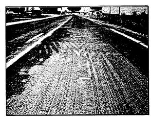
Photo of pavement surface after cold milling.
