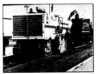
Photo of cold milling operation. Teeth mounted on rotating drum chip away material and feed it onto a conveyor belt for deposit into truck. The milled material is often reused (30 percent is common) in the rehabilitation of that or another pavement.
