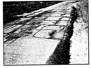
This photo shows an example of a failure caused by lack of drainage. Poor drainage can lead to numerous problems on both AC and PCC pavements.
