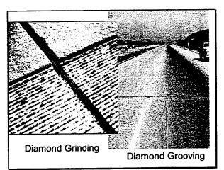
These photos illustrate the difference between a diamond-ground surface and a diamond-grooved surface.
