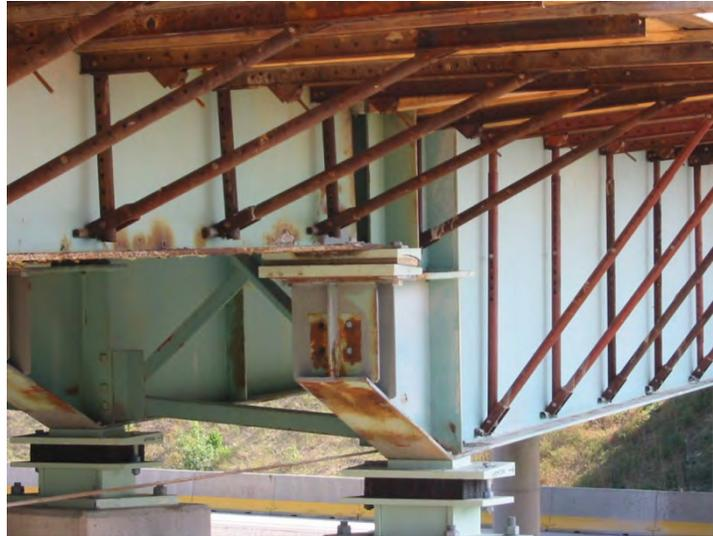
**Figure 6.3.2.6-1 Cantilevered Deck Overhang Brackets**
