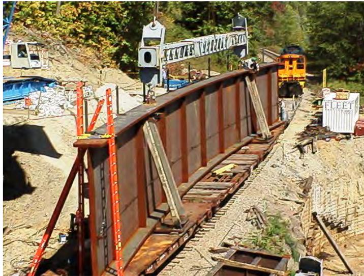
**Figure 6.3.2.4.2.2-1 Rail Shipment of a Steel Girder**
