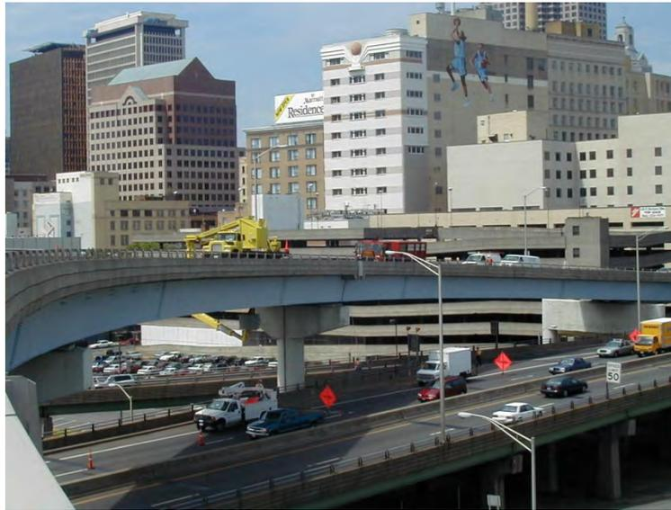
**Figure 6.3.2.3.1-1 Continuous-Span Steel Bridge**
