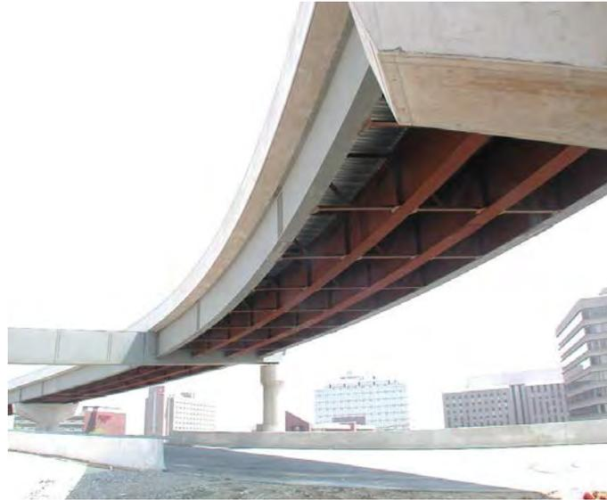
**Figure 6.3.3.3.3-1 Straddle Beam Supporting a Curved Steel I-Girder Bridge**
