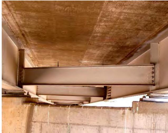
**Figure 6.3.2.9.5.1-4 Diaphragms in an I-Girder Bridge**
