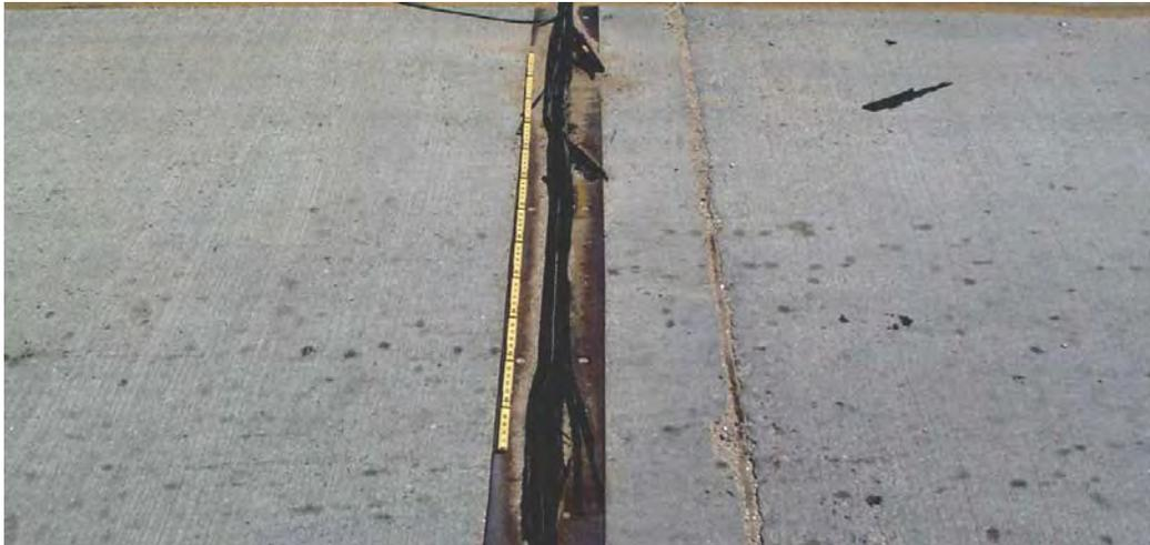
**Figure 2.3.2.1-1 Damaged Compression Seal Resulting in Leakage**
