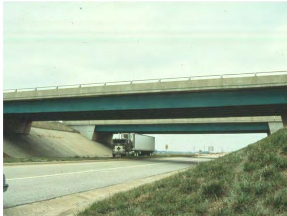
**Figure 6.3.2.12-2 Fabricated (Welded) Girder Superstructure**
