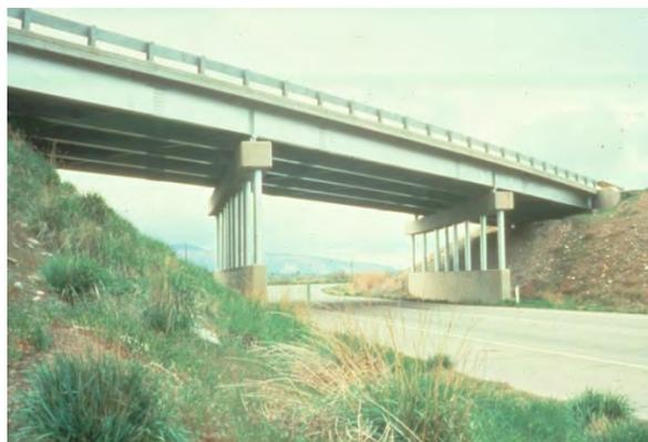
Figure 6.3.2.12-1 Rolled-Beam Superstructure
