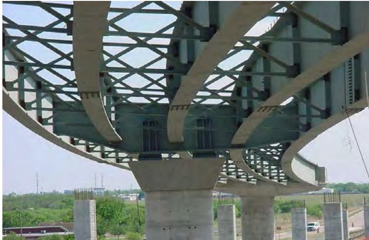
**Figure 6.4.9.2-1 Integral Steel Cap on a Curved I-Girder Bridge Without the Deck**
