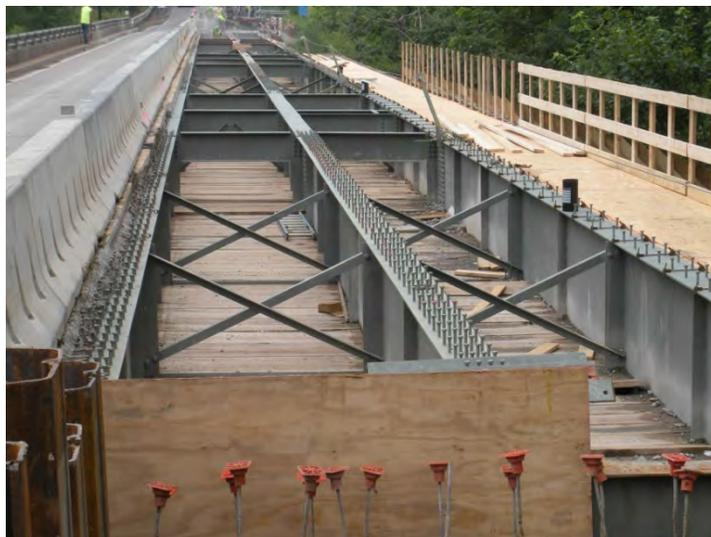
**Figure 2.3.2.3.1-2 Half-Width Redecking with Each Half on Three Girder Lines**
