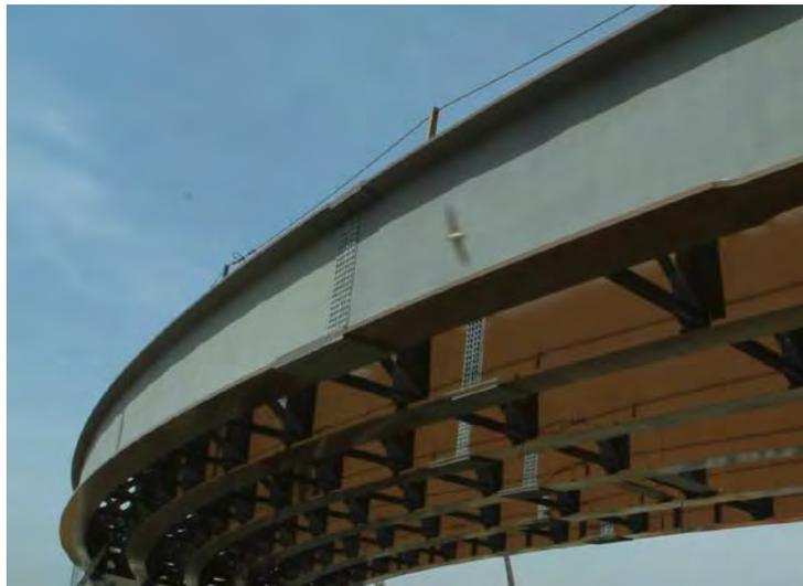
**Figure 6.6.5.1-1 Bolted Splice on a Curved Steel I-Girder**
