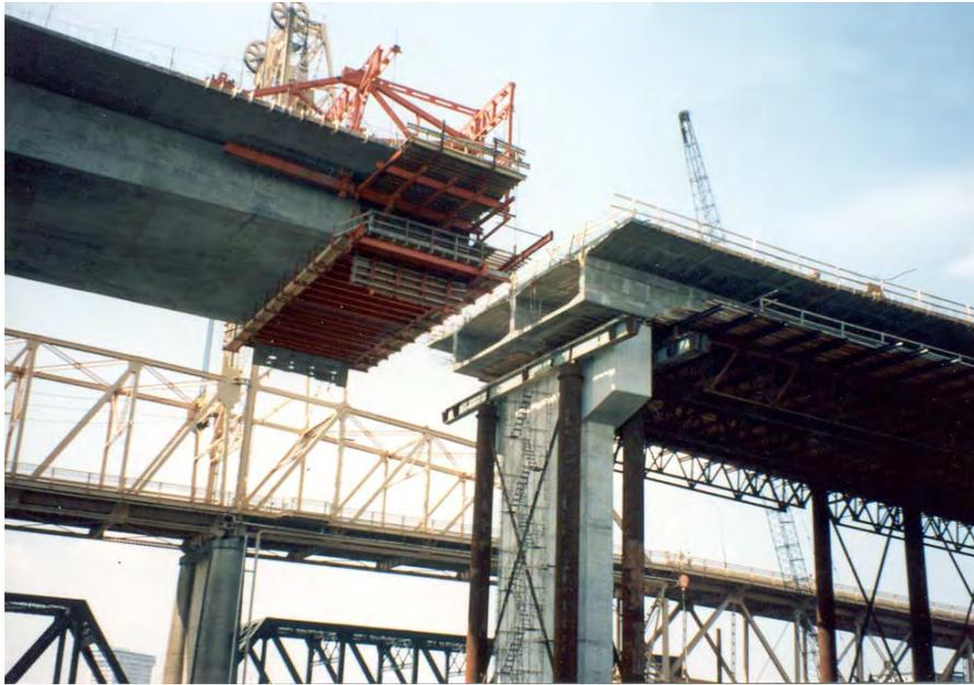
**Figure 5.10.6.2.1-1 Side-Span Falsework for Cast-in-Place Box (Acosta Bridge - Jacksonville, FL)**
