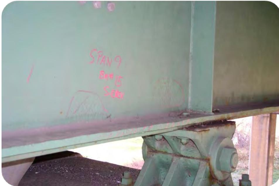
**Figure 6.6.6.3.1-1 Bearing Stiffener on I-Girder Web**
