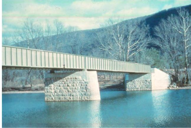
**Figure 6.3.2.5.8-2 Through-Type Two-Girder System**
