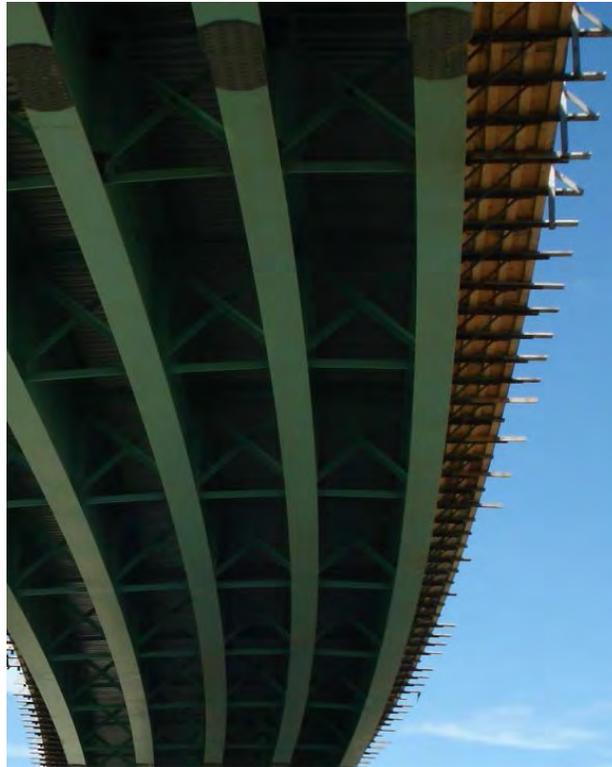
Figure 6.5.3.4.1-1 Overhang Brackets on a Curved I-Girder Bridge
