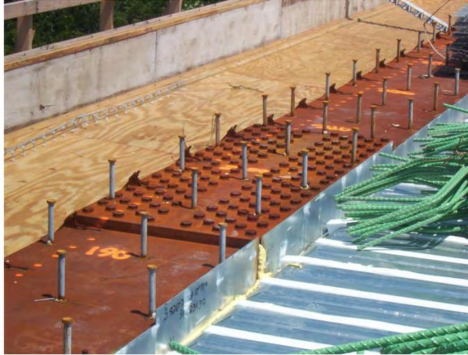
**Figure 6.4.2.1-1 Steel Girder with Stud Shear Connectors**
