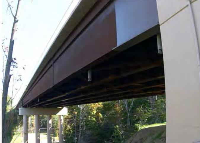
**Figure 6.4.5.5.2.2-1 I-Girder with Longitudinal Web Stiffeners**
