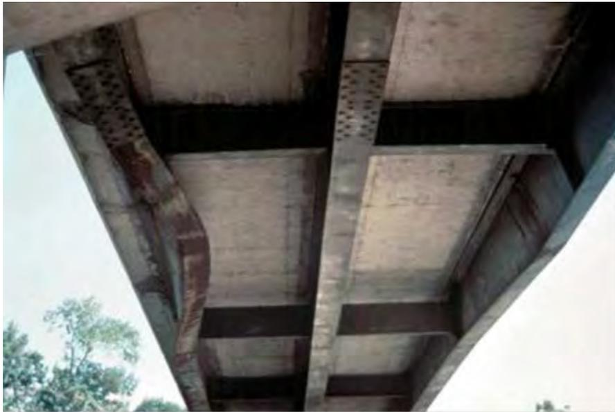
**Figure 2.2.3.2-1 Violation of Vertical Clearance Requirement**
