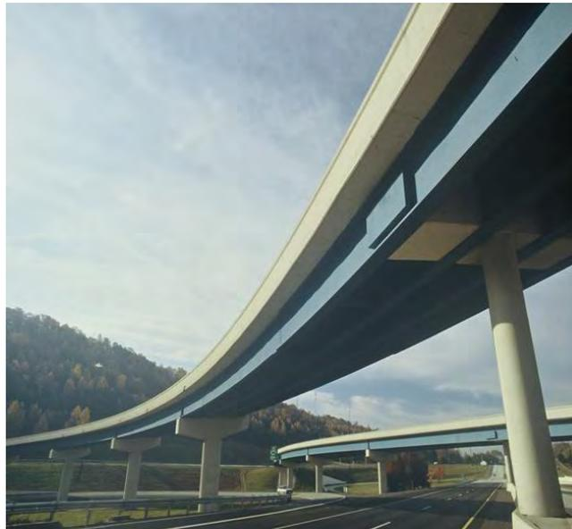
**Figure 6.3.3.3.4-1 Single-Column Integral Pier Cap**
