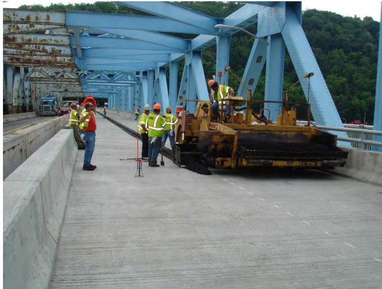
**Figure 2.3.2.3.1-1 Redecking Using Half-Width Construction**
