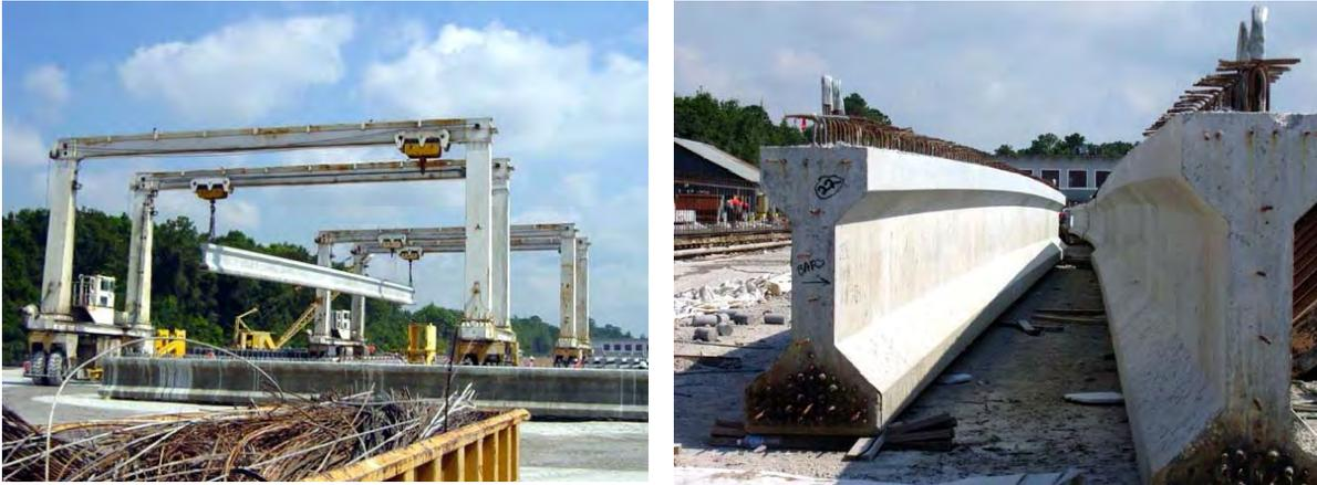
**Figure 5.2.1.4-1 Handling and Storage of Girders in Casting Yard**
