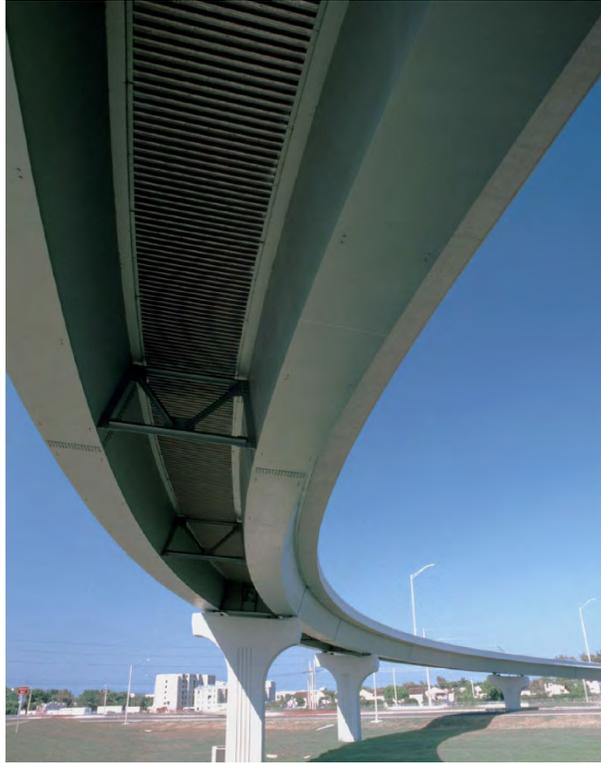
**Figure 6.3.2.11.2-1 Curved Steel Box-Girder Bridge**
