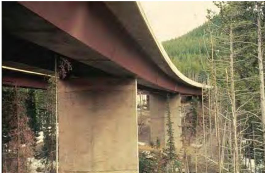
**Figure 2.2.1.1-1 Bridge with Curved Alignment**
