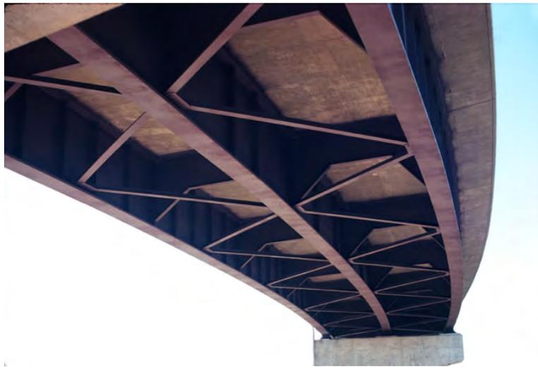
**Figure 6.3.2.10.2.1-1 Bottom Lateral Bracing on an I-Girder Bridge**
