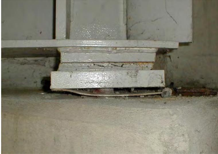
**Figure 4.2.3-1 Uplift on a Bearing**
