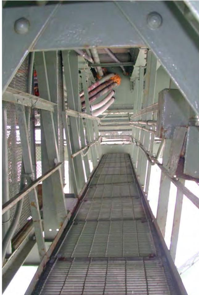
**Figure 2.3.2.2-1 Catwalk to Facilitate Bridge Inspection**
