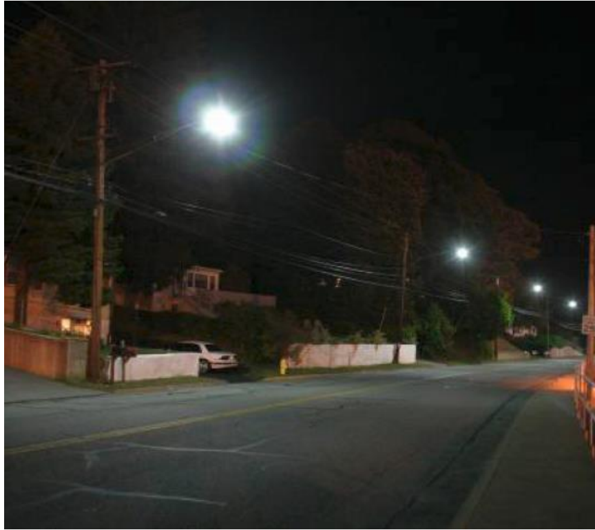
Electrodeless lamps used for street lighting.
