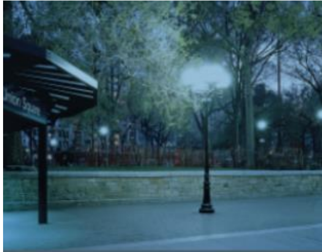
Induction lighting installed in Union Square Park in New York City.
