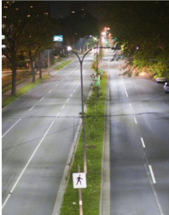
Luminaires in the median of this roadway provide uniform lighting on each side of the street.
