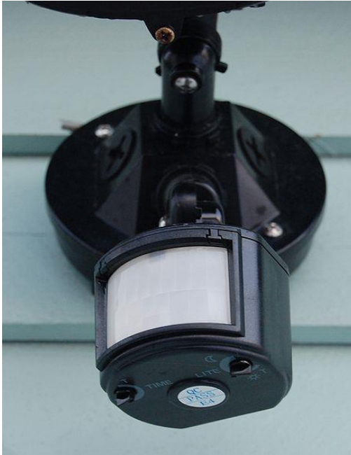
Left: An outdoor occupancy sensor. Right: An example of the field of view of an outdoor occupancy sensor.
