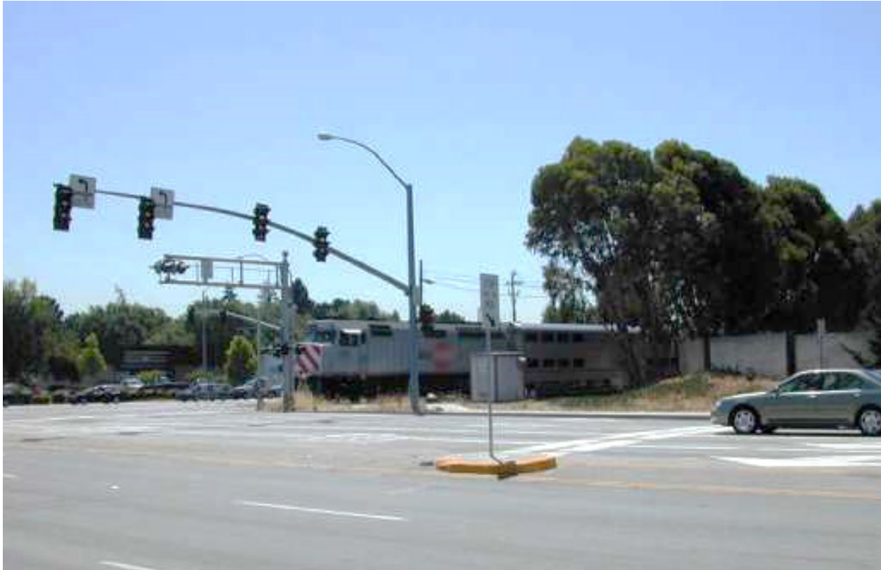
Figure 40. Illustrative Example Showing Displaced Stop Line (PCJX S. Mary Avenue Crossing at W. Evelyn Avenue, Sunnyvale, CA, USDOT 755037b)
