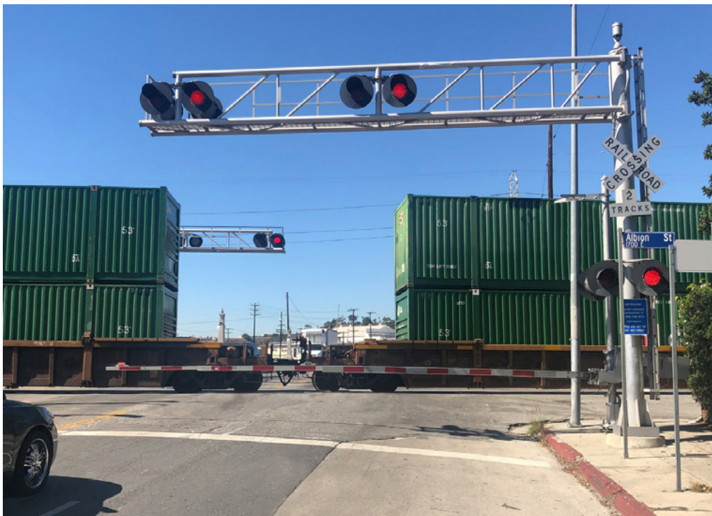
Figure 21. Illustrative Example Showing Cantilever with Flashing-Light Devices
