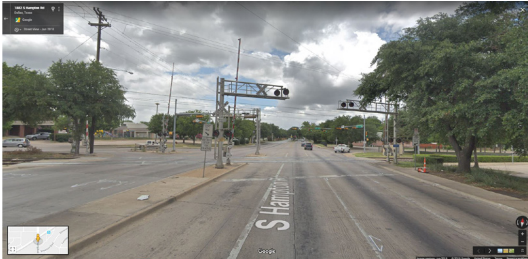
Figure 39. Illustrative Example Showing Use of Relocated Stop Line (Dallas Rapid Transit Red Line S. Hampton Rd Crossing at Wright Street, Dallas, TX)
