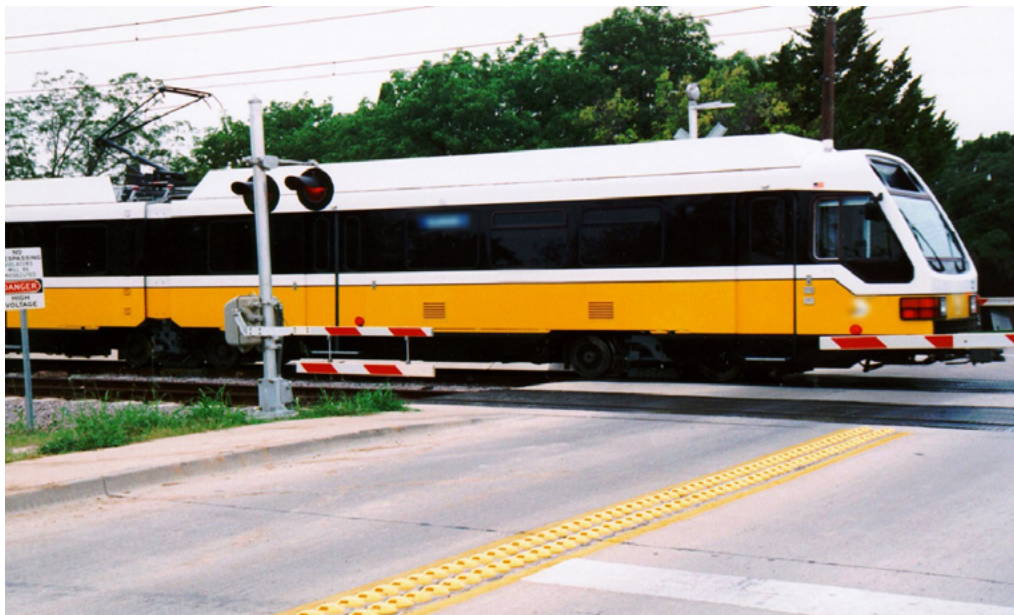
Figure 60. Illustrative Example of Pedestrian Gate with Skirt (DART Blue Line Lynn Haven Avenue Crossing, Dallas, TX)
