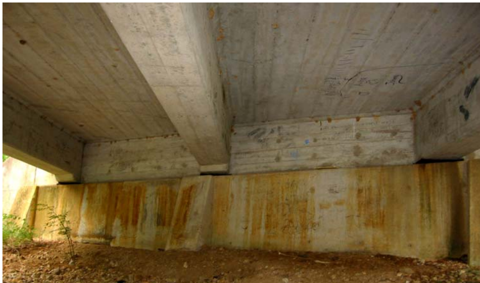
Figure 3.10. Bridge X-495 Substructure
