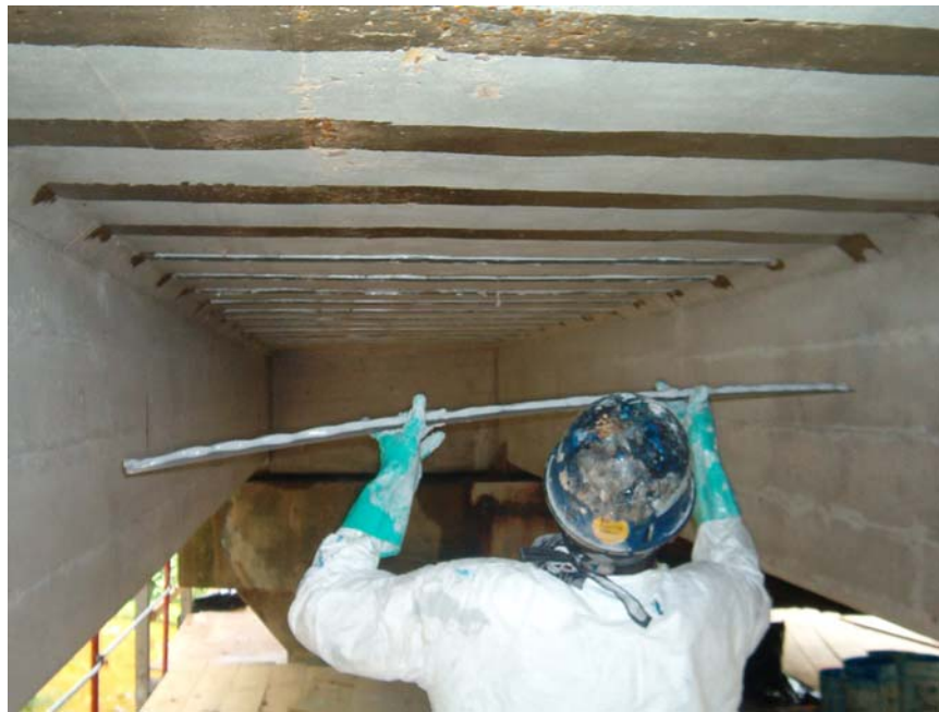
Figure 2.2. Pre-cured Laminate FRP Installation
