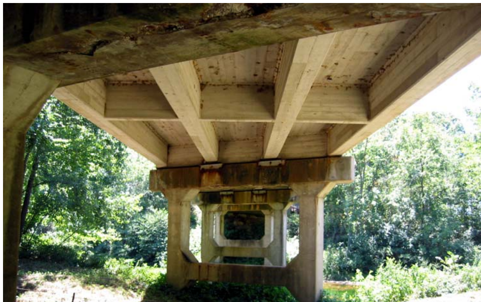
Figure 3.8. Bridge T-530 Substructure
