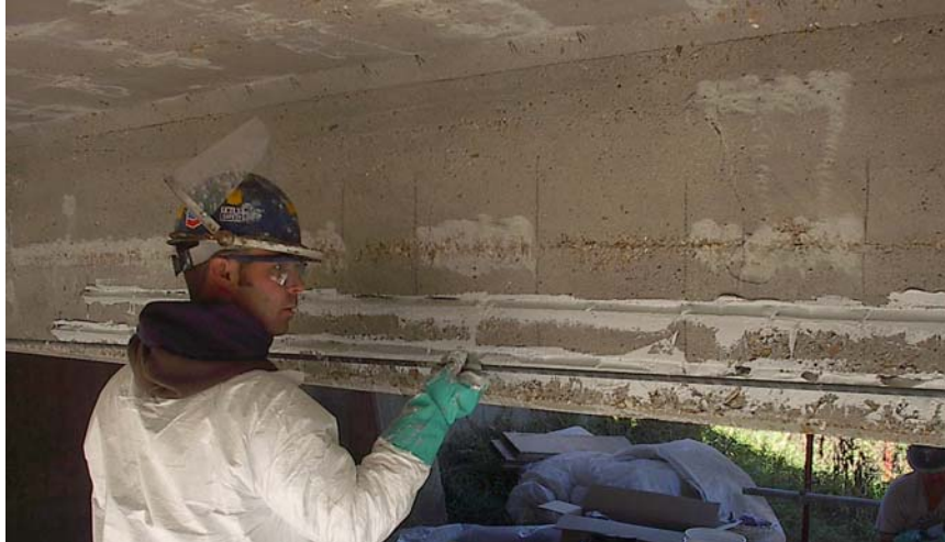
Figure 2.3. NSM Bar Installation
