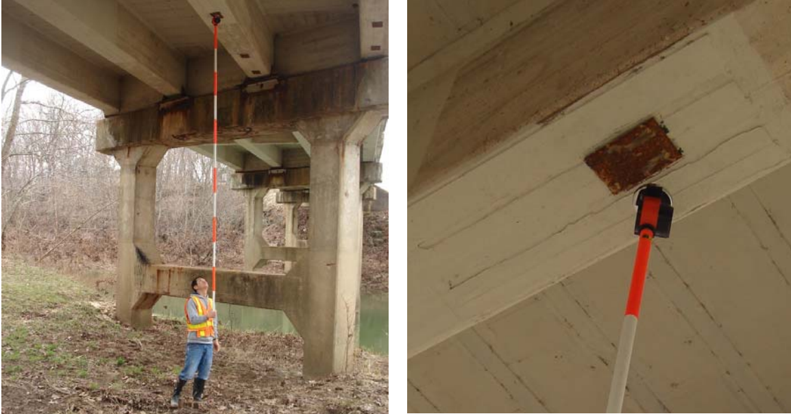
Figure 5.3. Attaching Target Prisms with Range Pole
