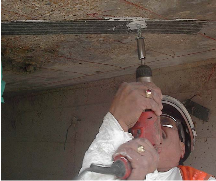
Figure 2.5. MF FRP Installation
