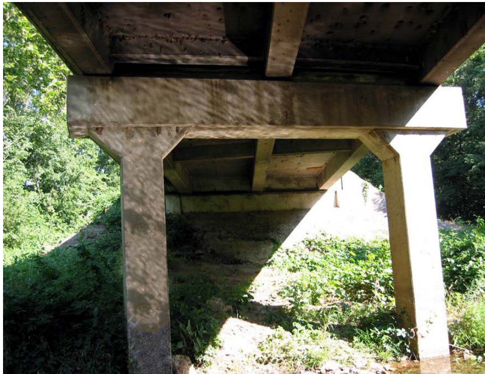
Figure 3.12. Bridge P-962 Substructure
