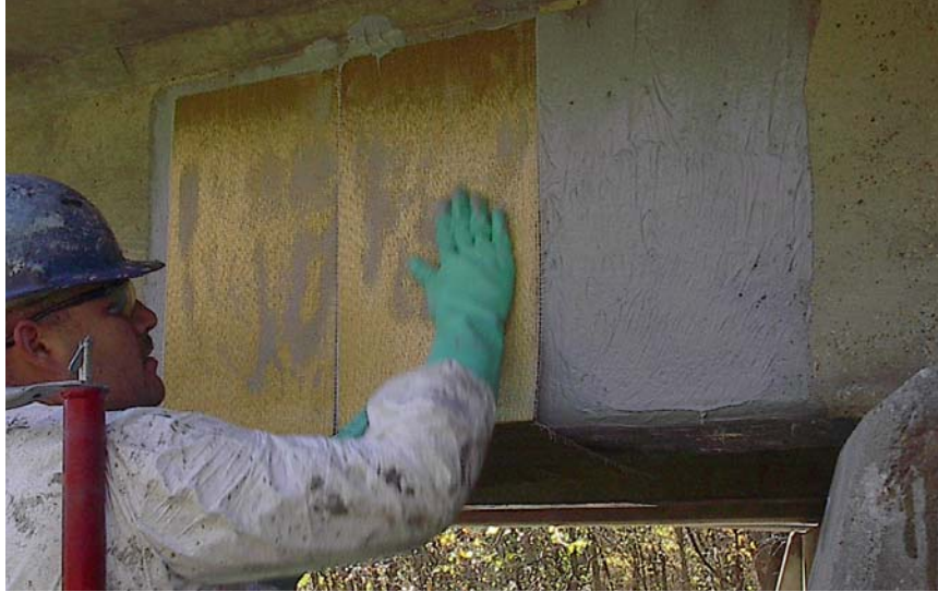
Figure 2.4. SRP Installation Bridge P-962
