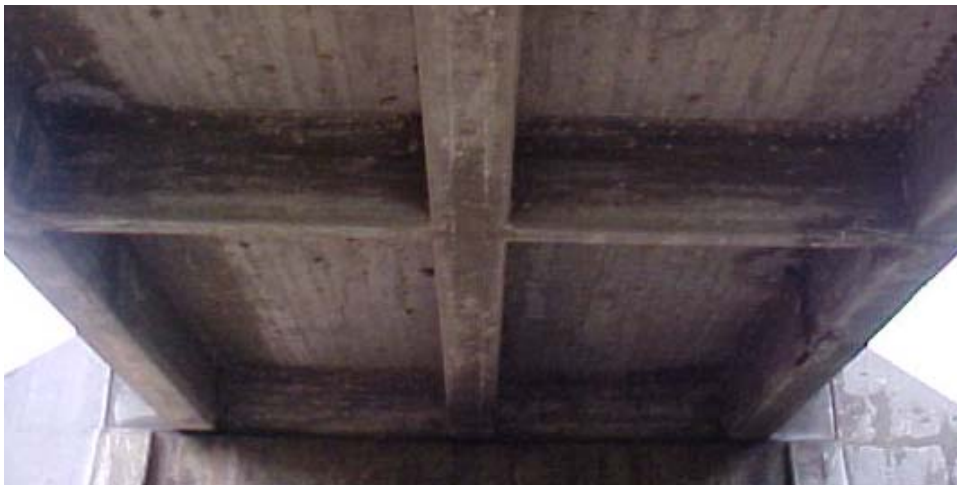
Figure 3.3. Bridge X-596 Superstructure
