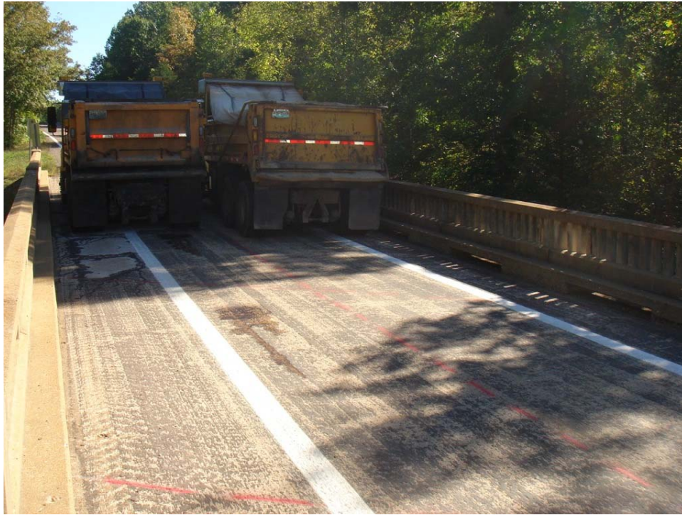
Figure 6.4. Bridge X-495 Shading of Deck During Testing
