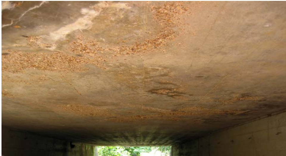
Figure 3.14. Bridge Y-298 Substructure
