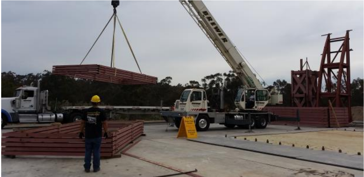
Figure A-1: Transportation of the laminar frames to the shake table
