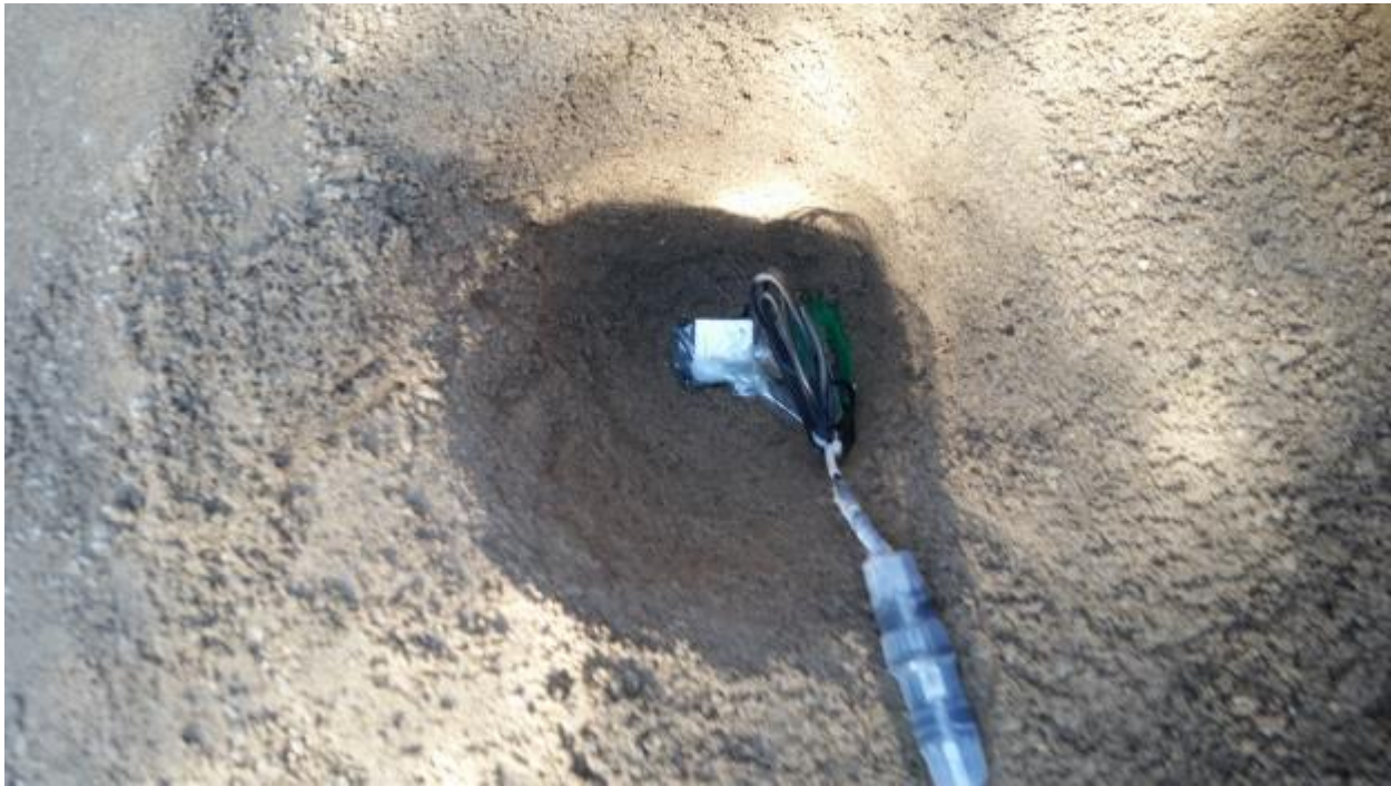
Figure A-10: Placement of accelerometer during backfilling
