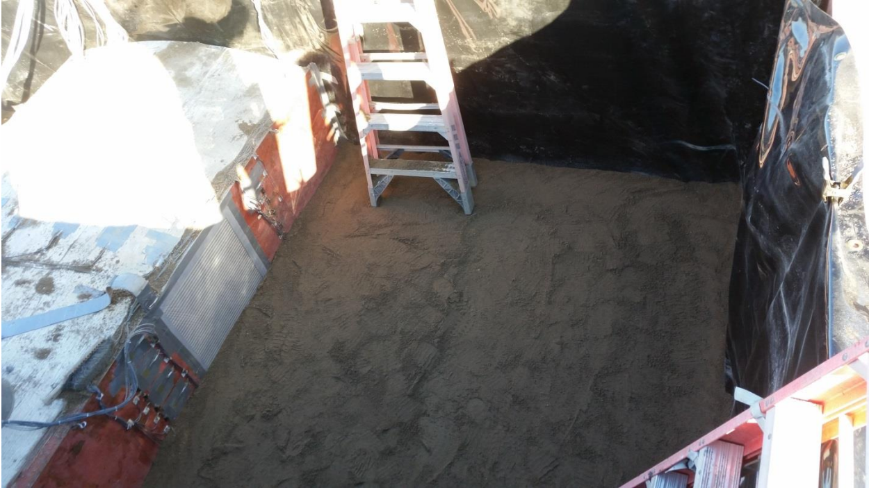
Figure A-12: Backfilling
