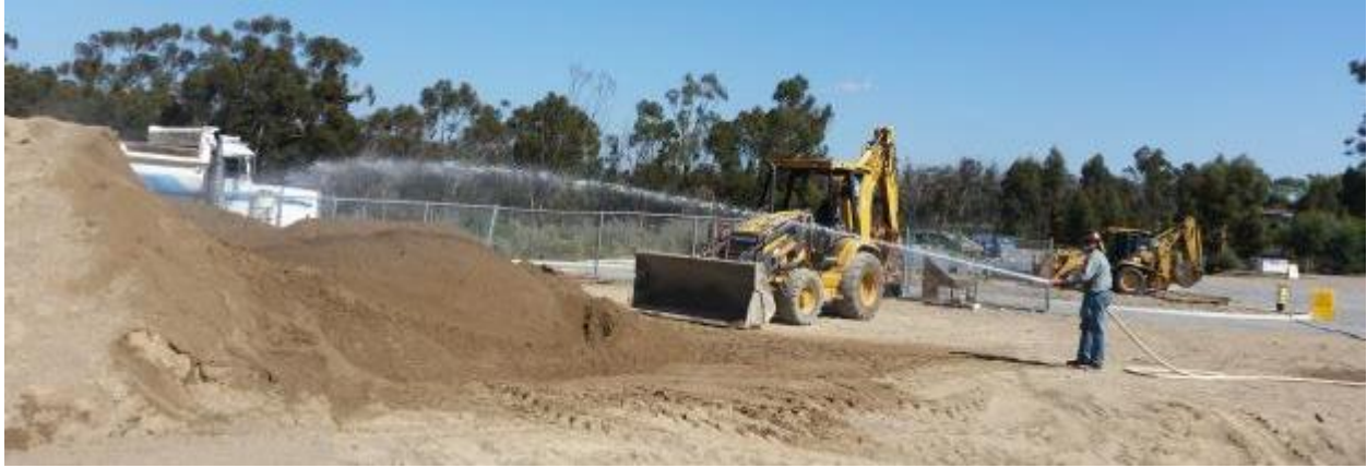
Figure A-5: Adjusting soil moisture
