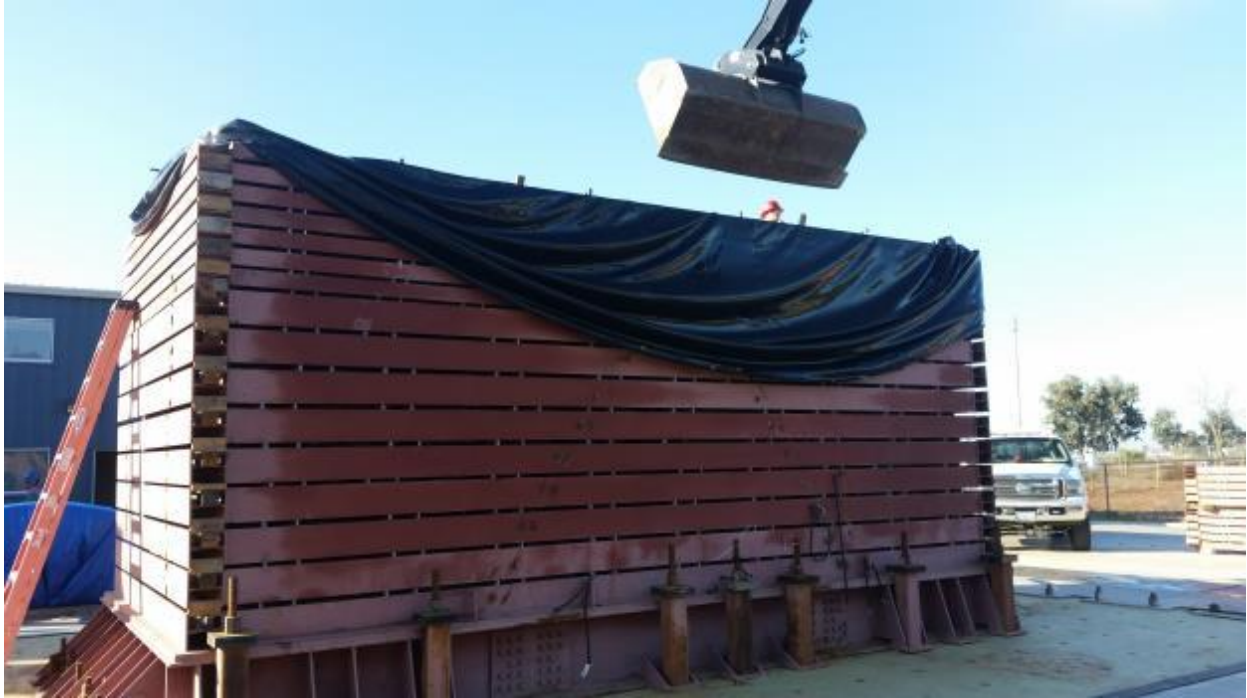
Figure A-7: Backfilling
