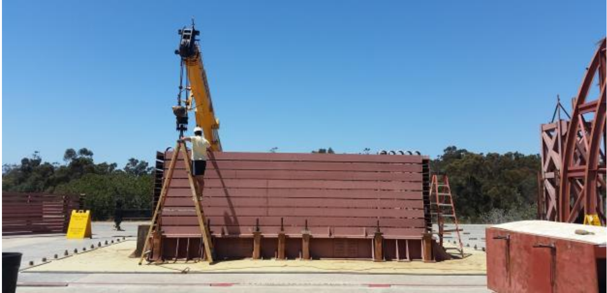
Figure A-3: Assembly of the laminar soil container frames
