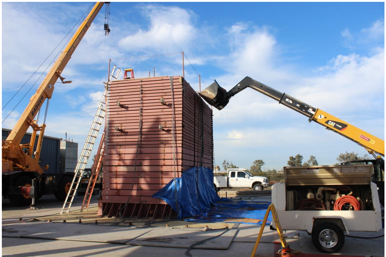
Figure A-13: Replacement of backfill
