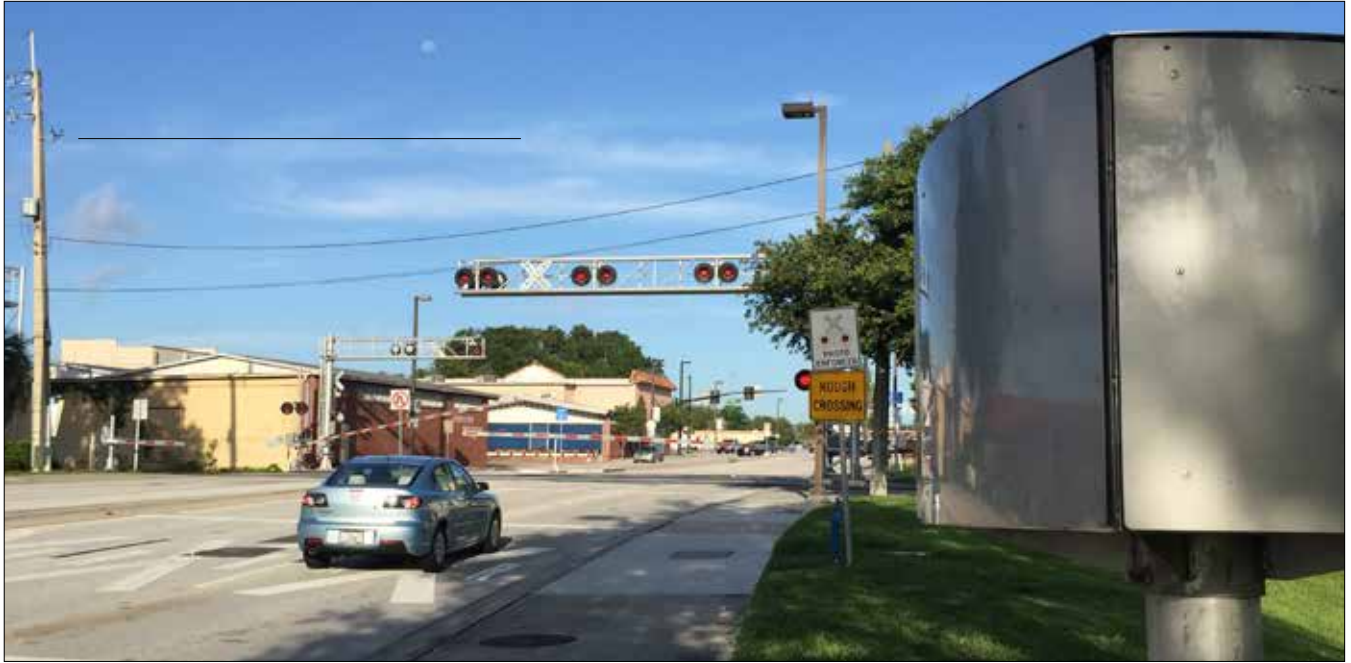
Above: Photo enforcement system installed at the East Princeton Street grade crossing in Orlando, Florida. Source: U.S. DOT Volpe Center
