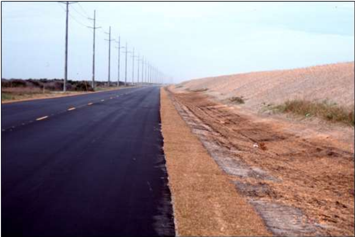
Figure 5-11. Artificial sand dune constructed seaward of North Carolina Highway 12 to protect the roadway from flooding and damage (FHWA 2008).
