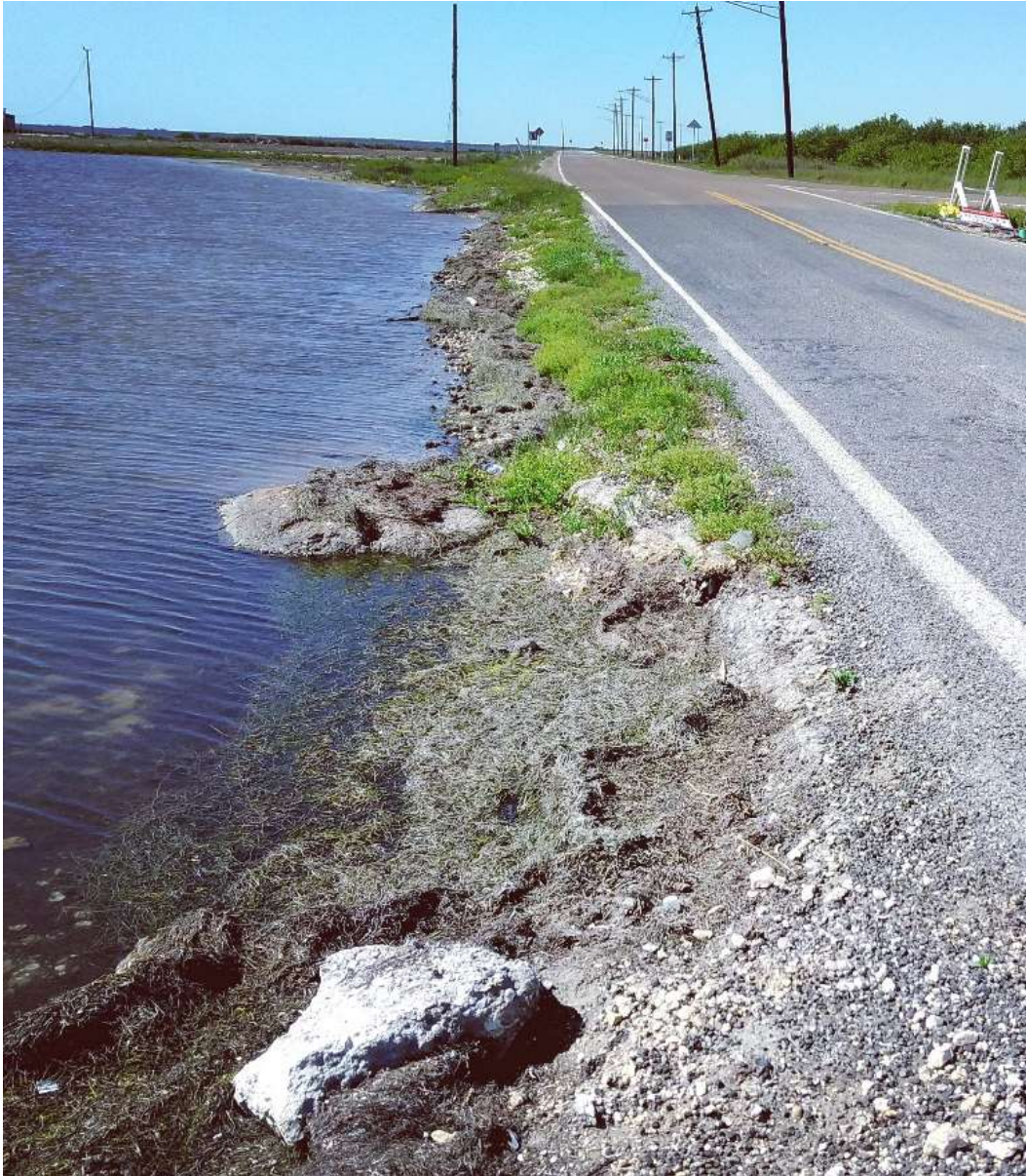
Figure 4-7. Laguna Shores Road under typical (non-storm) conditions. Note the irregular edge of pavement and proximity to open water (photo courtesy of Corpus Christi MPO).
