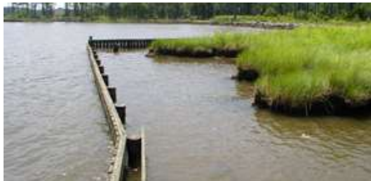
Figure 5-3. Vertical timber sill protecting a marsh (NCDEQ 2019).
