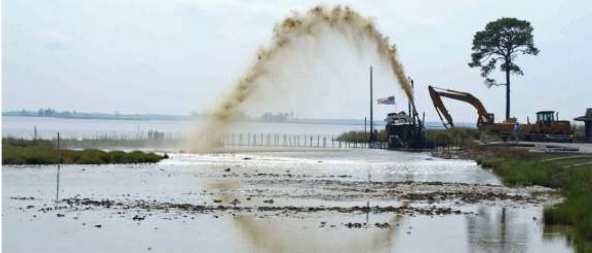
Figure 2-2. Thin layer placement of dredged material (photo courtesy of USACE 2019b).
