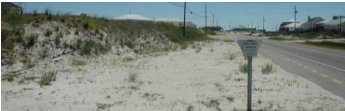
Figure 2-1. A constructed, vegetated dune protects this low-elevation barrier island roadway during storm events (photo courtesy of Bret Webb).
