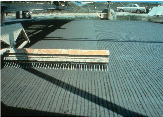
Figure 13. Transverse tining operation and resulting surface texture.
