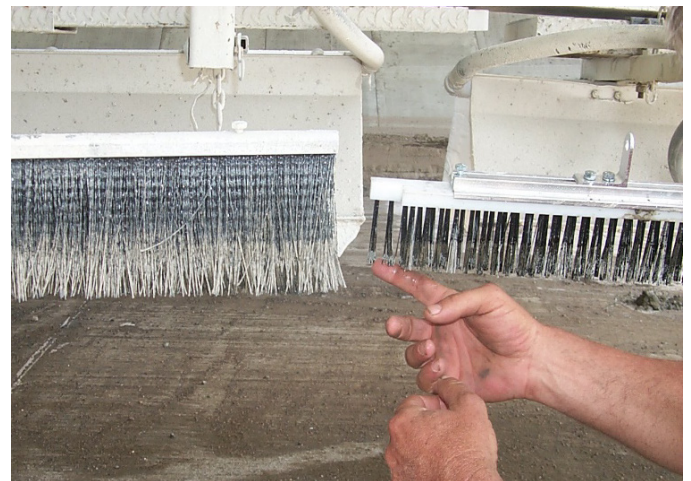
Figure 14. Typical mechanical brooms and resulting concrete pavement texture.
