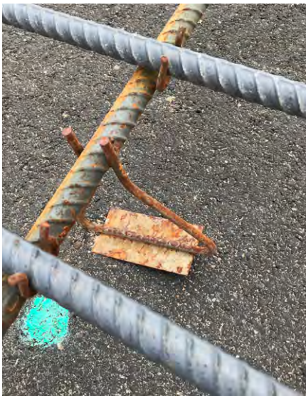
Figure 5. Transverse bar support system.
