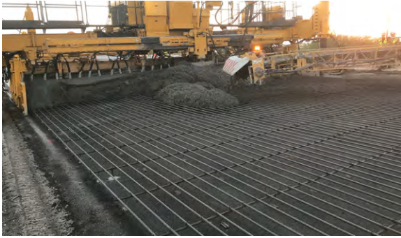
Figure 9. Concrete being discharged in front of the slipform paver.
