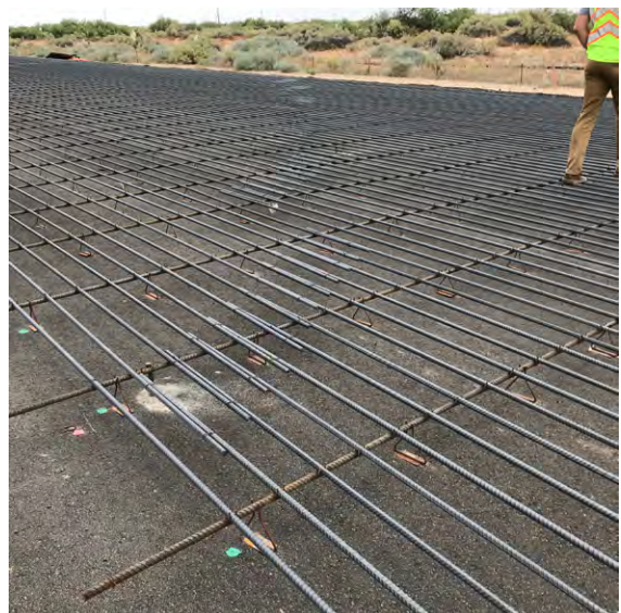
Figure 8. Longitudinal bar splicing.
