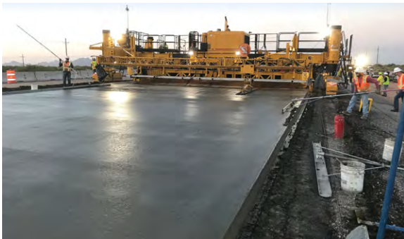
Figure 10. Finishing operation behind the paver.
