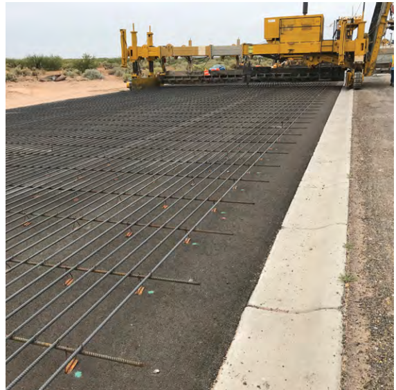
Figure 7. Steel reinforcement placed over the AC base.
