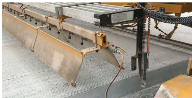
Figure 12. Curing operation and use of side nozzle.
