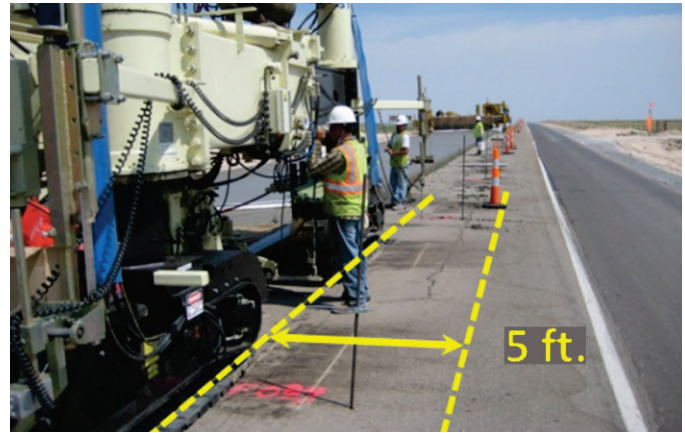
Figure 1. Operating space requirements for conventional paving (ACPA 2013).
