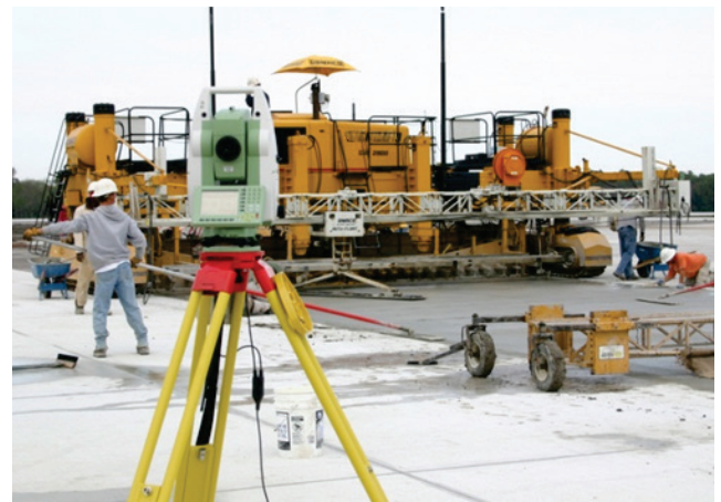
Figure 5. Robotic total station in use on a project site (ACPA 2013). © 2013 ACPA
