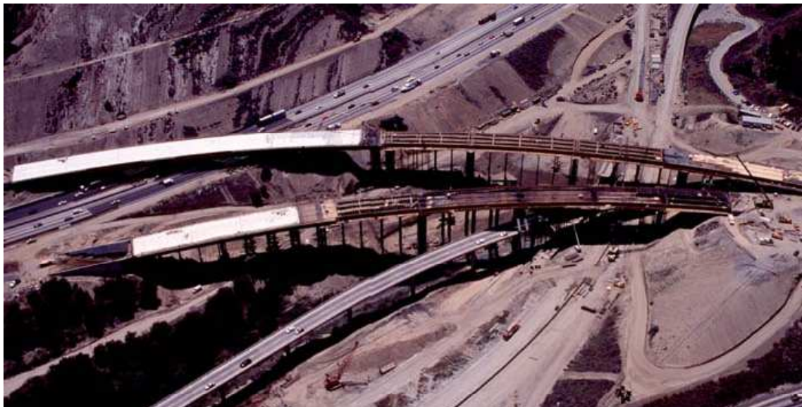
Figure 17. Reconstruction after the Northridge earthquake (Source: Caltrans)
