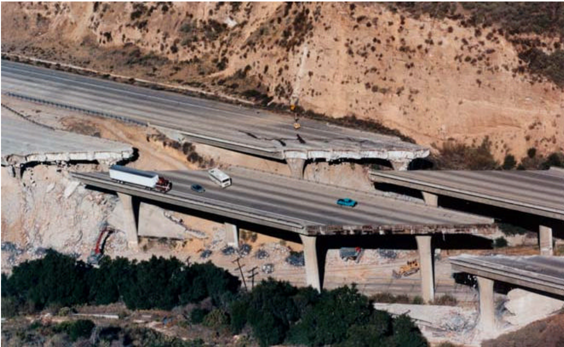
Figure 11. I-5 damage at Gavin Canyon
