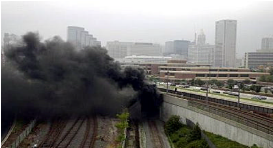
Figure 8. Smoke from the south portal of the Howard Street Tunnel
