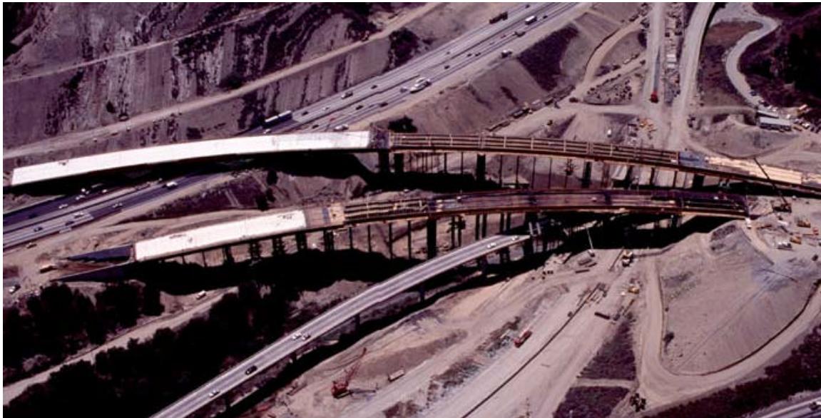
Figure 14. Reconstruction after the Northridge earthquake
