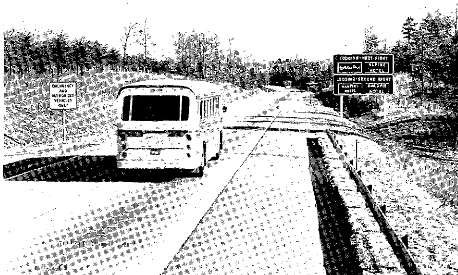
Signing is a vital factor in highway safety. Shown: Experimental signing on I-95 in Northern Virginia tests driver reaction.
