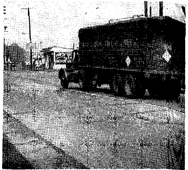
Fig. S - Section of concrete on left was laid in 1915, near Easton, Pa.
