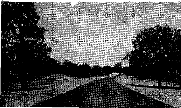
THIS TEXAS ROAD TYPIFIES DESIGN FOR TRAFFIC OF NOT OVER 1,000 VEHICLES A DAY Pavement Is 24 Ft Wide, with Wide Shoulders and Easy Slopes
