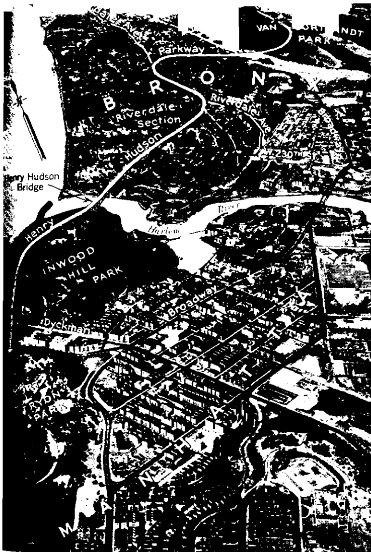
AERIAL VIEW OF PARKWAY PROJECT FROM SOUTHERN END
