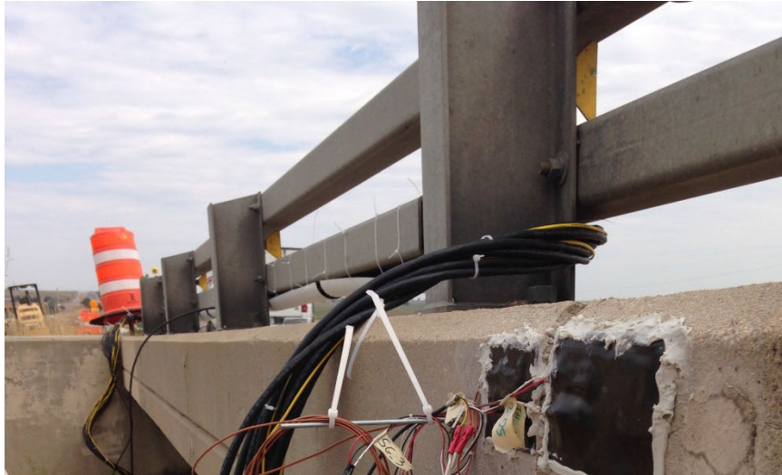
Figure 3.27 Wires along railing
