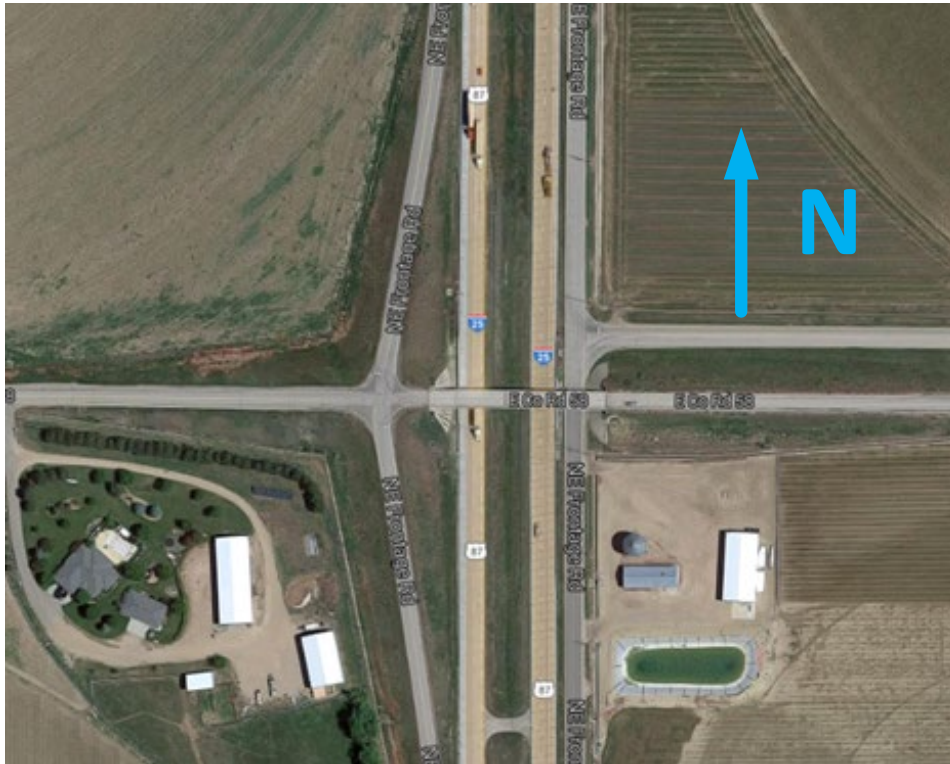
Figure 3.1 Plate Girders for Bridge B-16-FM (Google Maps Image)
