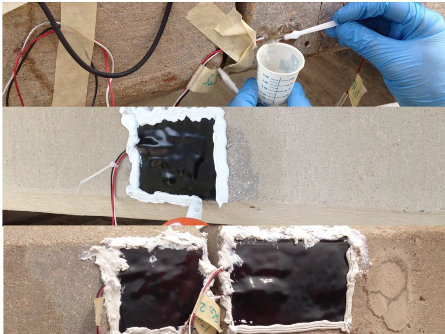
Figure 3.16 Strain gauge protection
