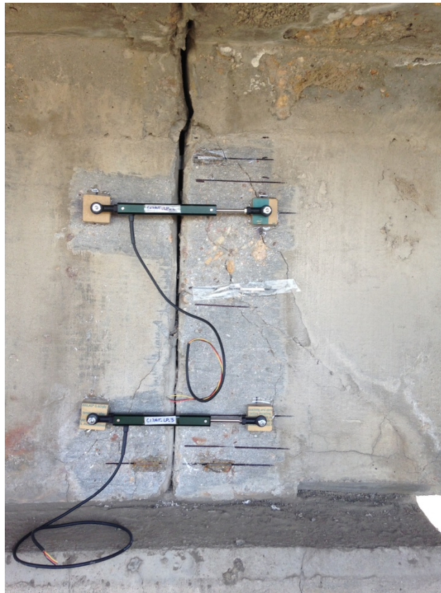
Figure 3.21 Linear potentiometer in place on joint
