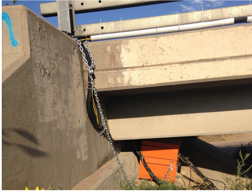
Figure 3.25 Job box on north abutment
