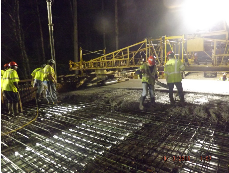
Figure 5. Bridge Construction Showing Nighttime Deck Concrete Placement
