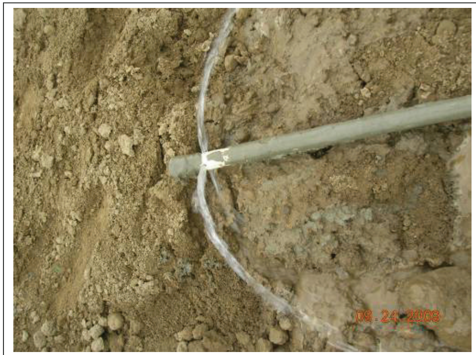
Figure 3. Photograph. Outlet end of flushing tube.
