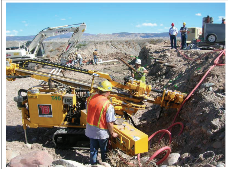
Figure 10. Photograph. Casing installation at the Sunset Mesa Site.
