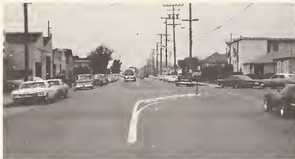
Figure 45. Forced turn channelization — Berkeley, CA.
