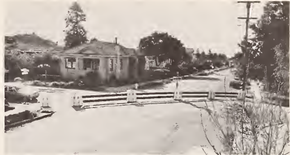
Figure 11. Temporary diagonal diverter — Berkeley, CA.
