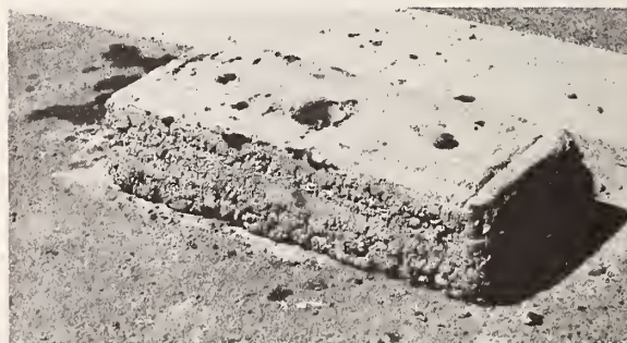
Figure 10. Typical undercarriage barrier in diverter's emergency vehicle gap
