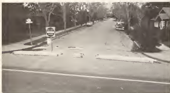
Figure 21. Temporary cul-de-sac — Palo Alto, CA.
