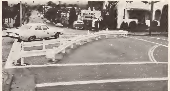
Figure 14. Diagonal diverter — Berkeley, CA.
