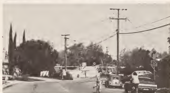
Figure 7. Rumble strip installations — for neighborhood speed control.
