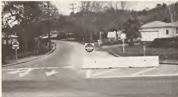
Figure 36. Semi-diverter — Walnut Creek, CA.
