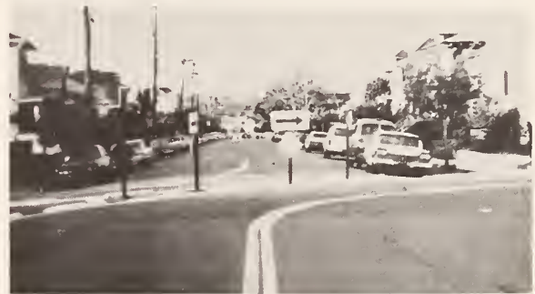
Figure 8. Temporary diagonal diverter — Berkeley, CA.
