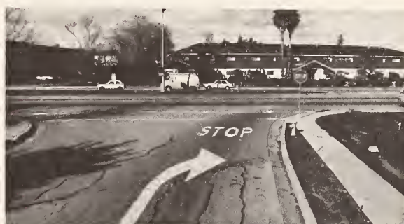
Figure 48. Median Barrier — Redwood City, CA.
