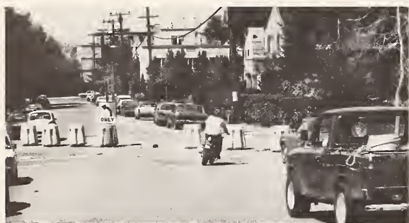
Figure 9. Temporary diagonal diverter — Berkeley, CA.
