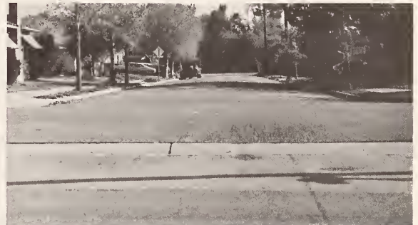
Figure 69. Transverse Valley Gutter — Redwood City, CA.
