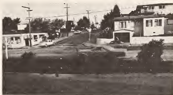
Figure 47. Median Barrier — Albany, Ga.
