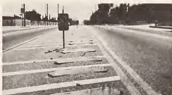
Figure 49. Median Barrier — Los Angeles, CA.
