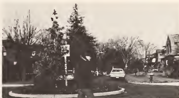
Figure 56. Permanent Traffic Circle — Seattle, WA.
