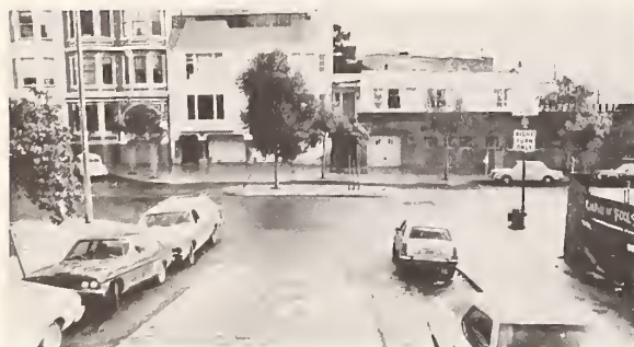
Figure 46. Forced turn channelization (ineffective design) — San Francisco, CA.
