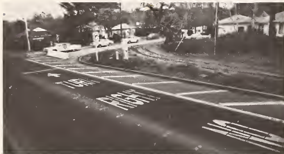
Figure 37. Semi-diverter treatment — Walnut Creek, CA. (Note evidence of avoidance route on lawn at right)
