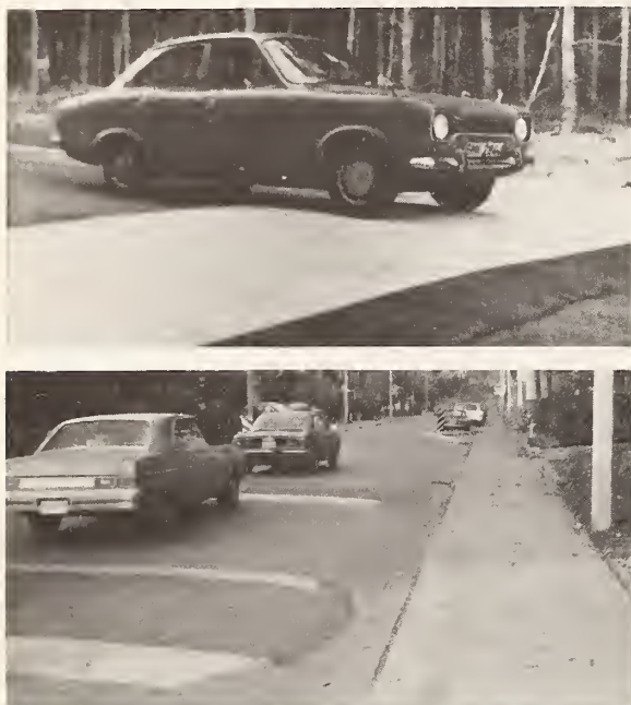
Figure 5. British speed undulation. In Toronto (lower view) undulations have been deployed in pairs.
