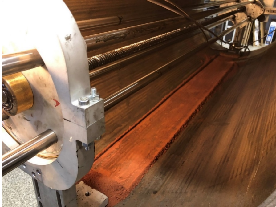
Figure 62. A photo showing the ferrite oxide powder at the bottom of the pipe.
